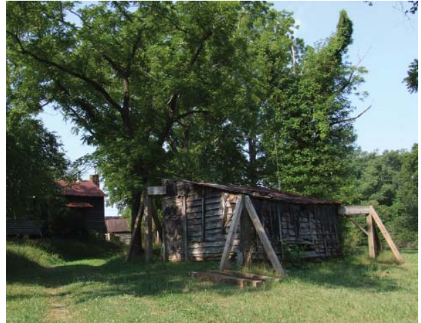
Figure 140. View southwest of Brood House.
