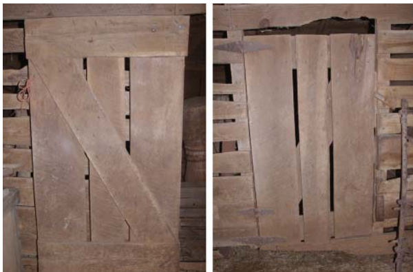
Figure 88. View of door at center crib on west side.
