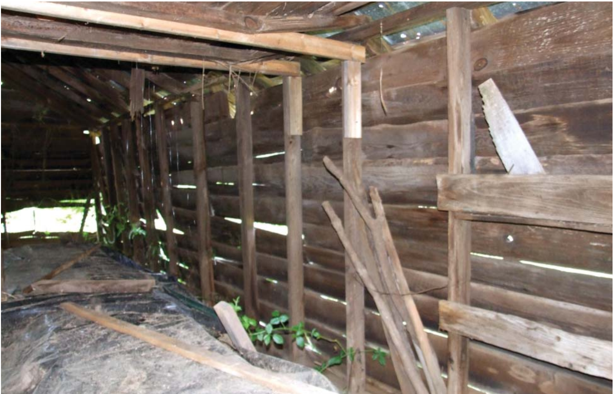
Figure 66. View southwest in west addition to the Barn.
