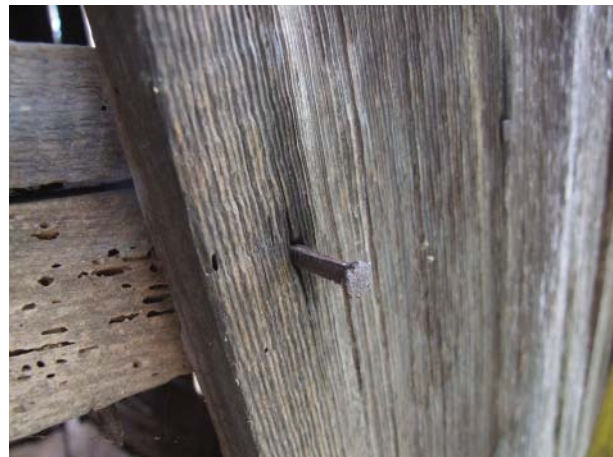
Figure 6. View of typical nineteenth-century cut nail on the Old Corn Crib.
