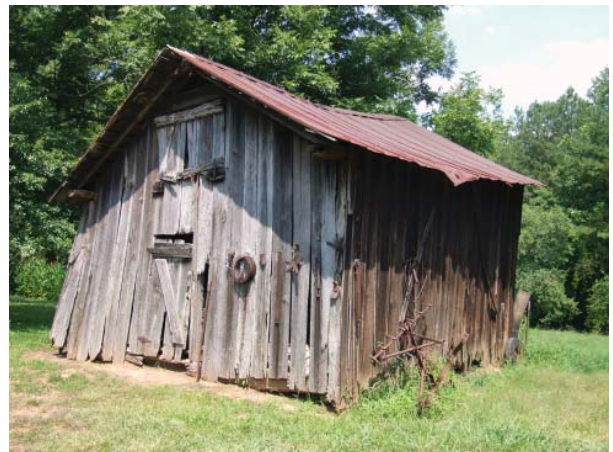
Figure 25. View of Old Corn Crib in 2008, prior to stabilization..
