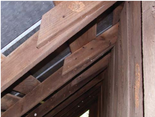
Figure 72. View of typical rafter tails on original barn.
