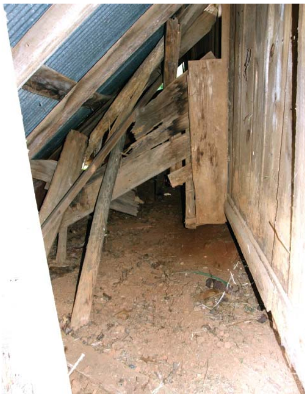
Figure 69. View south in second east addition.
