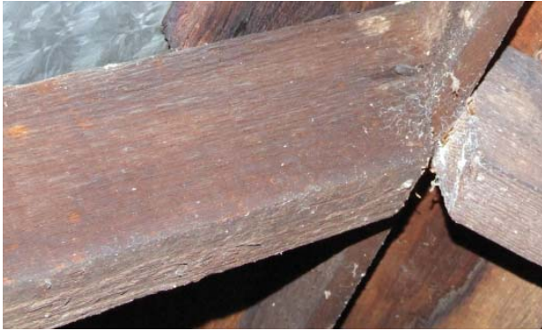
Figure 2. View of rafter in roof of the log pen of the main house. The vertical saw marks characteristic of the early reciprocating saws are visible on the rafter at left.
