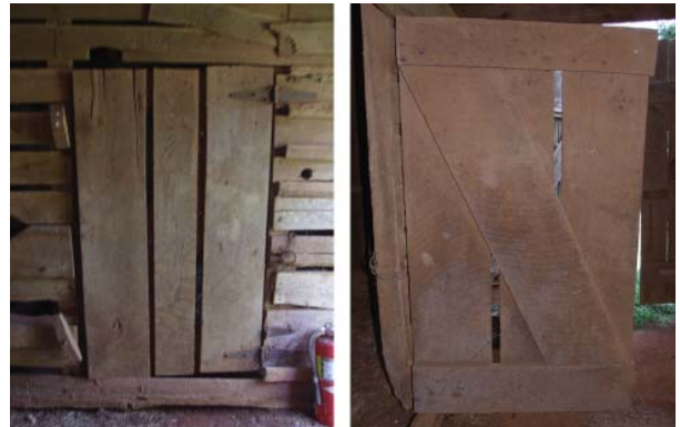
Figure 90. View of door at northwest crib.
