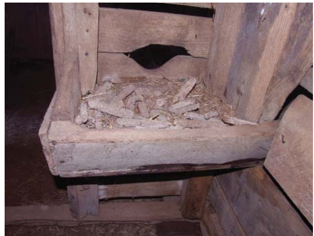
Figure 99. View of trough in northeast crib, a continuation of the trough in the middle west crib.
