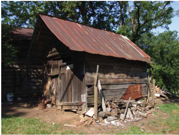
Figure 19. View of Gear House in 2008.
