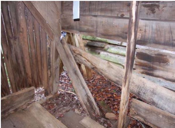
Figure 36. View of southeast corner of Gear House where sills have been completely destroyed.
