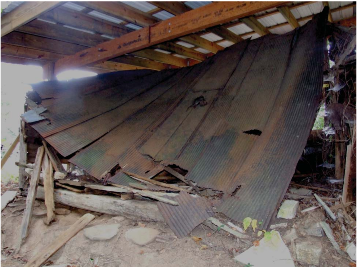
Figure 127. View of collapsed rear (north) side of Goat House.
