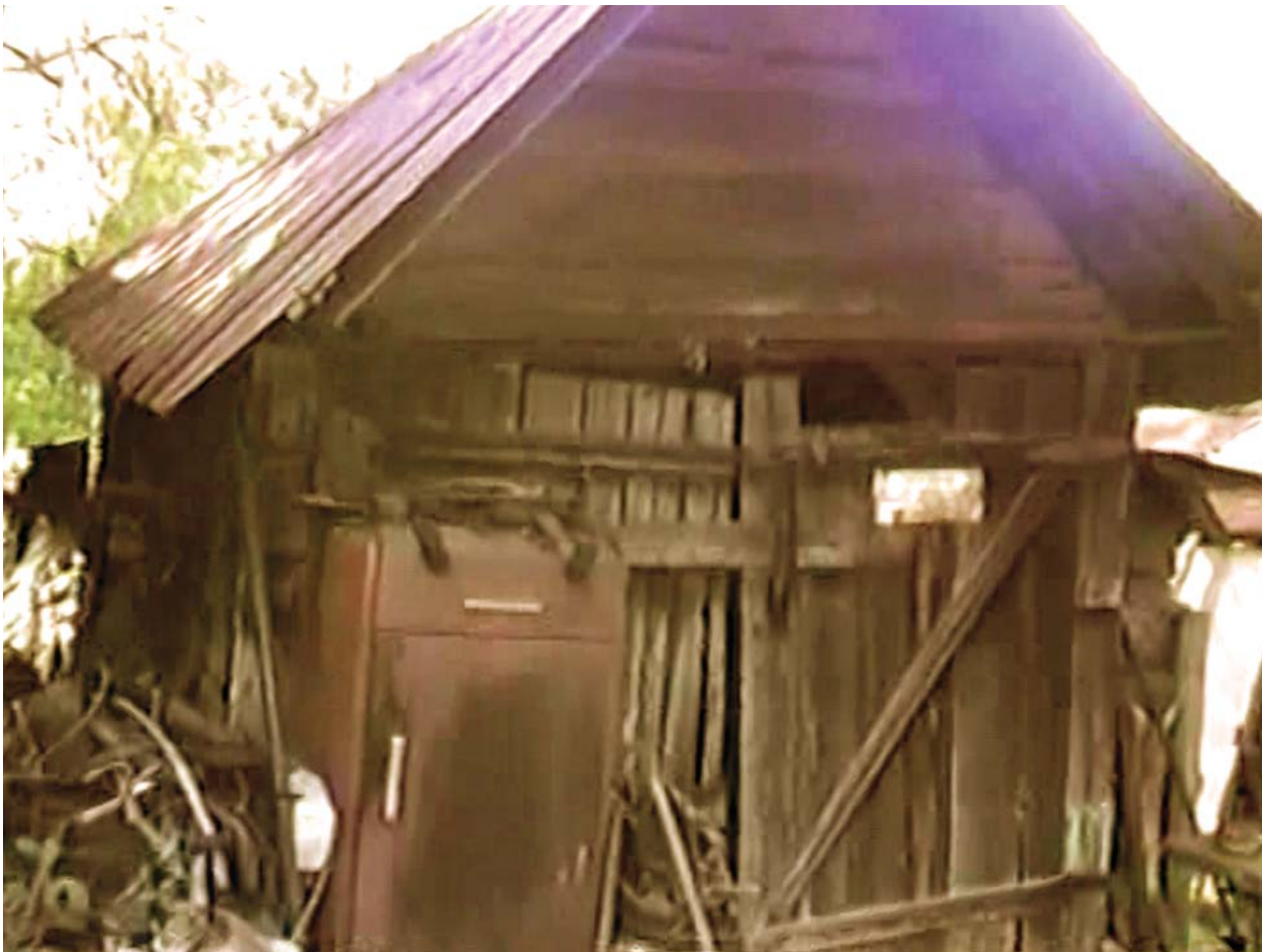
Figure 20. View of Gear House in the 1970s. (Shirley Gaddis Jordan Collection)
