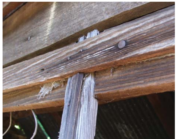
Figure 135. Detail of window cover at front opening, with remnants of string-reinforced polyethylene sheeting visible beneath the battens used to attach it to the frame.
