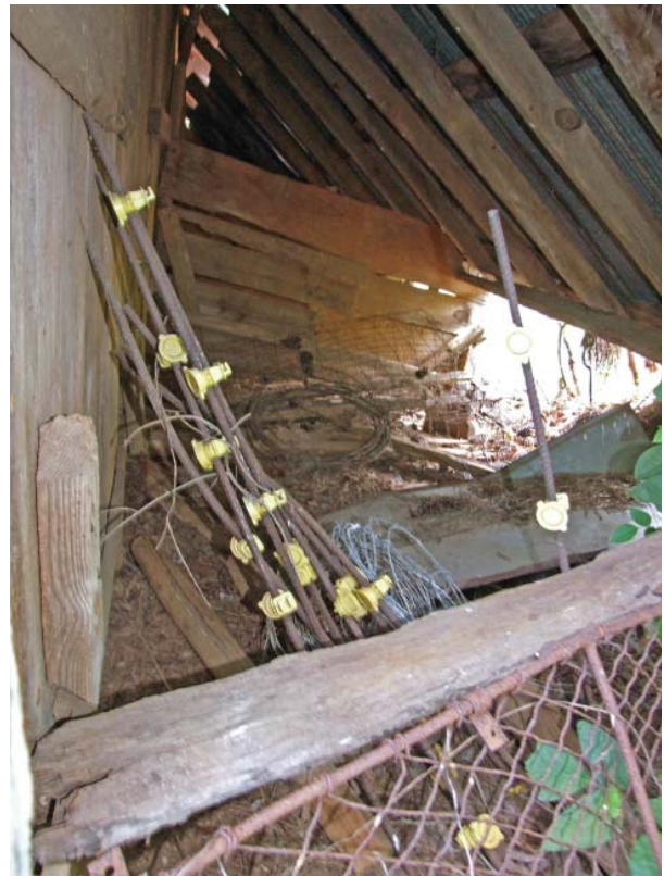
Figure 70. View north in second east addition.
