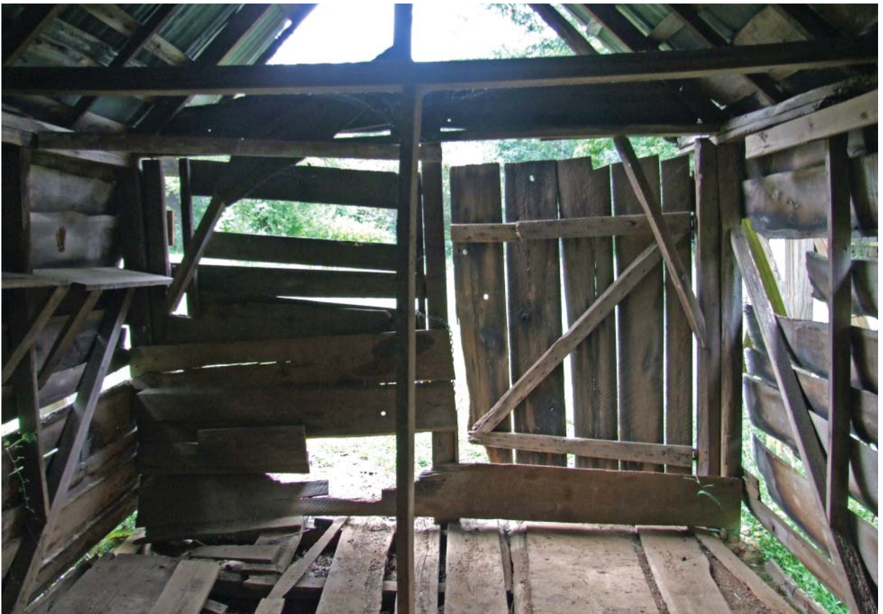
Figure 22. View east inside Tool Shed.
