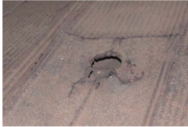
Figure 131. View of hole in roofing for stove flue.
