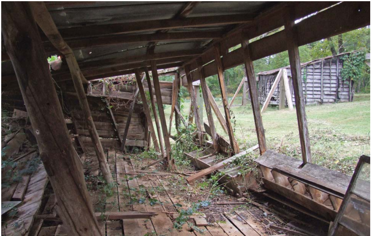
Figure 156. View east in North Chicken House.
