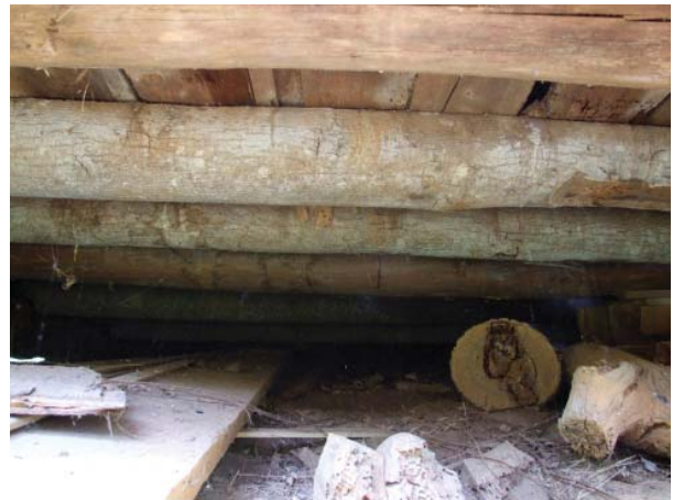
Figure 52. View west under Old Corn Crib.
