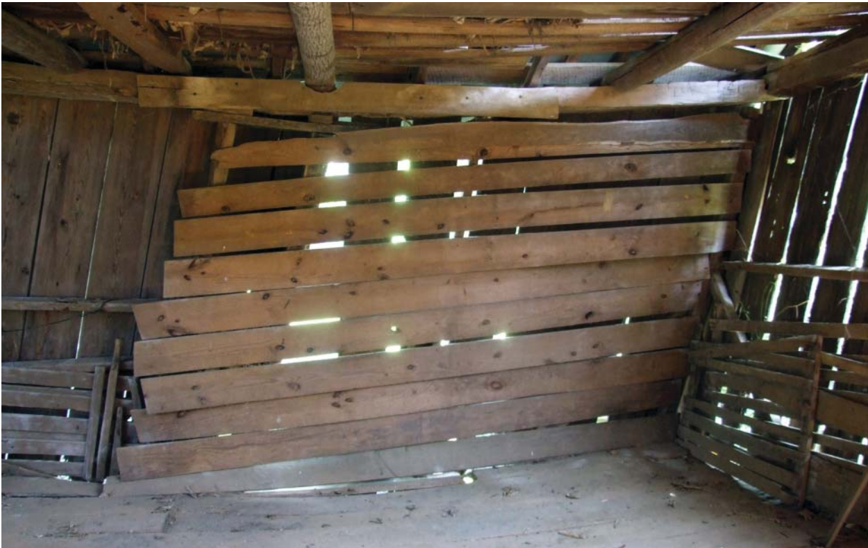
Figure 50. View of north wall of Old Corn Crib.
