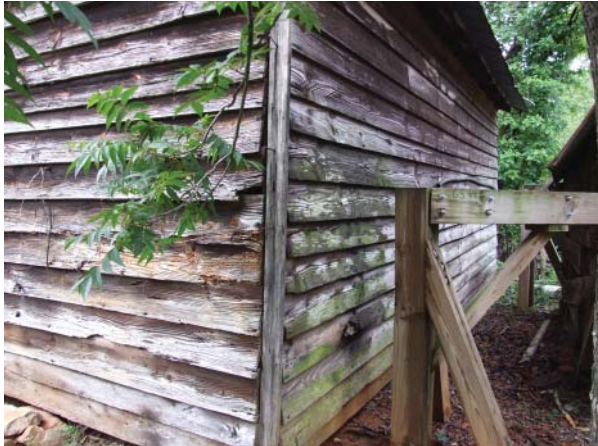
Figure 114. View west of northeast corner of corn crib.
