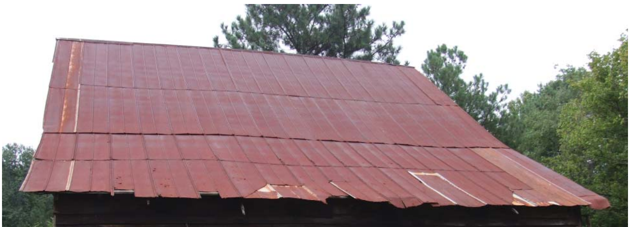
Figure 106. View of roofing on west side of the Barn.
