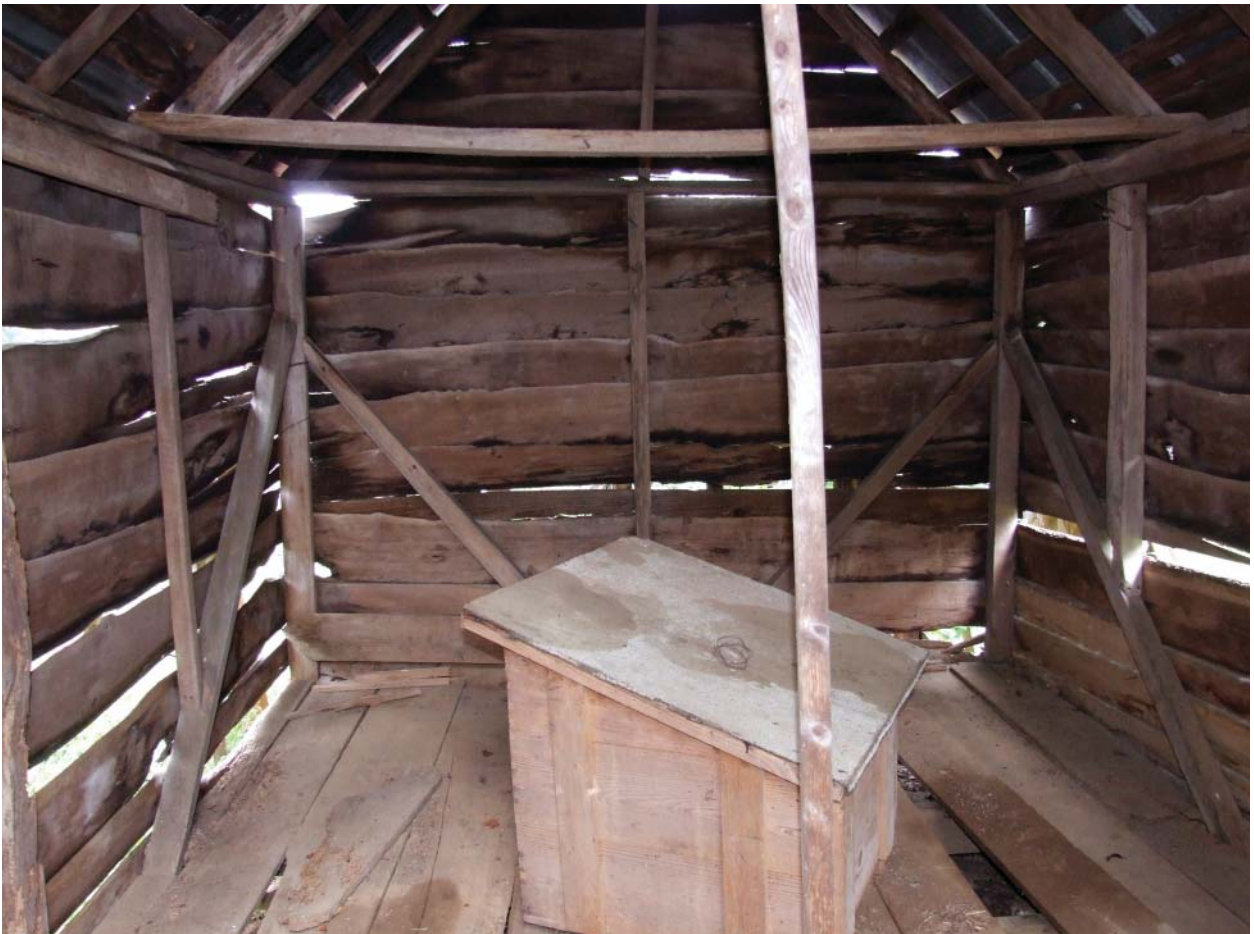
Figure 17. View west in Tool Shed.
