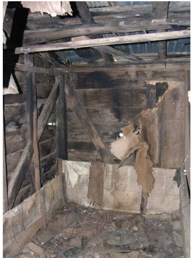
Figure 147. View of northwest corner of Brood House
