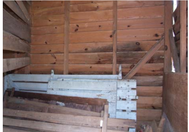
Figure 116. View north of east end of corn crib.
