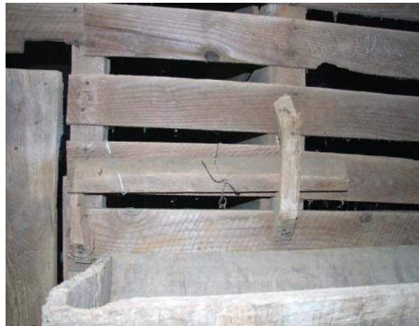
Figure 96. View of sliding bar latch for southwest crib door.
