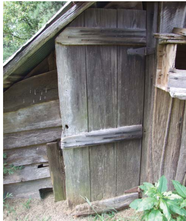
Figure 86. View of door at north end of second east addition.
