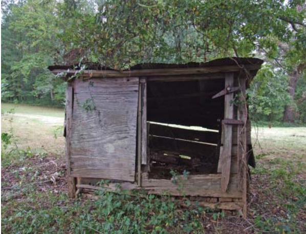
Figure 166. View of front (west) side of Hog House.
