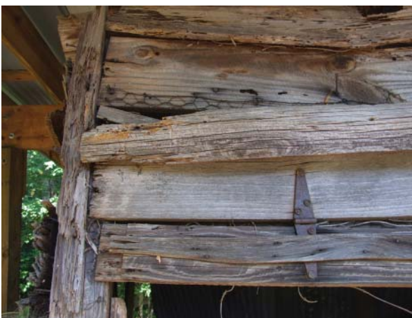
Figure 133. View at southwest corner of Goat House, showing top rail and hinge for window cover. Remnants of chicken wire are visible at what may have been the original top of the opening.
