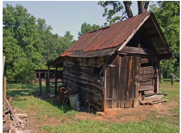
Figure 18. View of Tool Shed in 2008.
