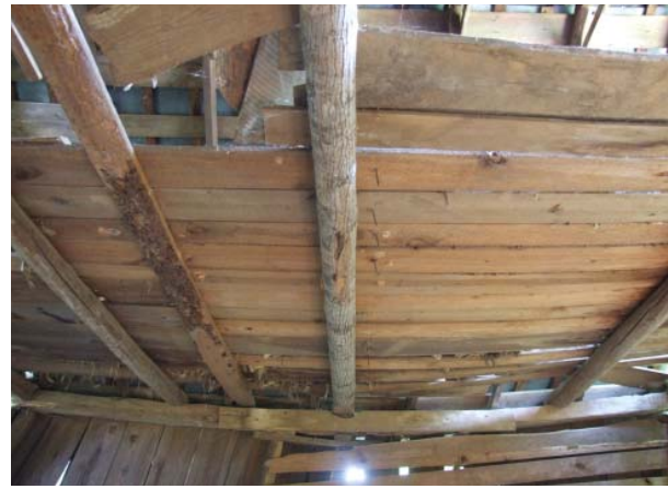
Figure 46. View of joists and flooring for loft.
