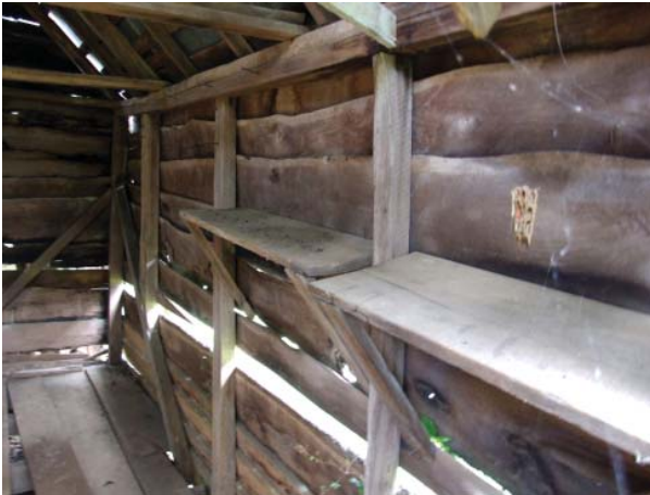
Figure 21. View of north wall of Tool Shed.
