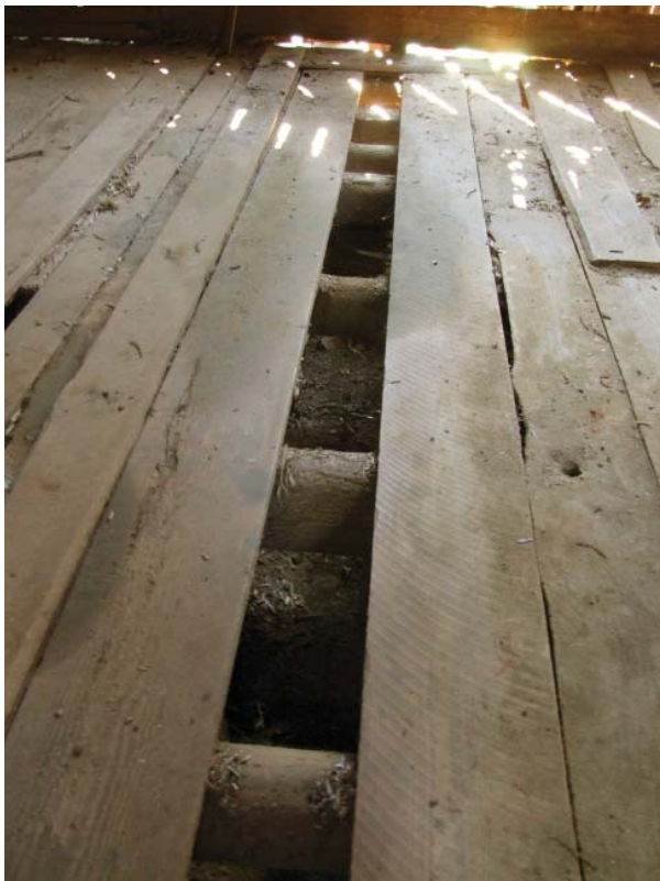
Figure 51. View of flooring in Old Corn Crib, with one piece removed to show log joists.
