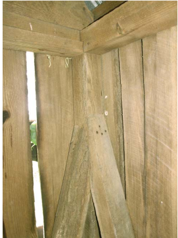
Figure 71. View of intersection of corner post, braces, and wall plates at southwest corner of the original barn.
