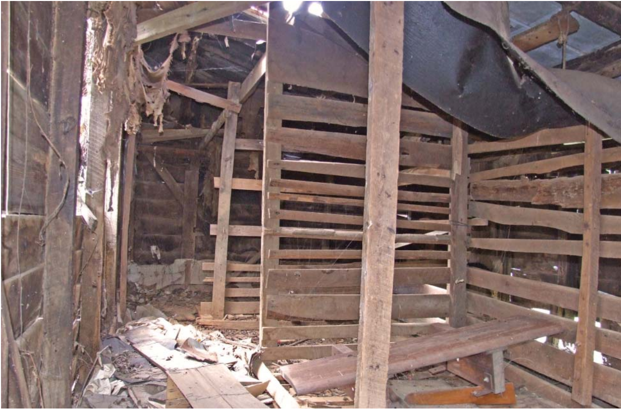
Figure 145. View west inside Brood House.
