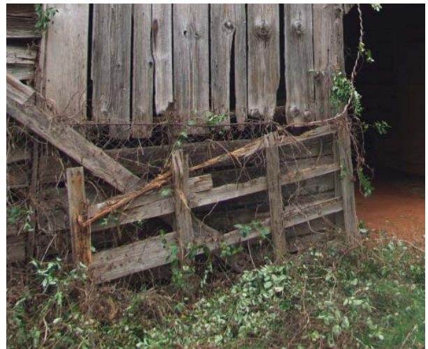
Figure 82. View of gate at south end of center aisle in 2008.
