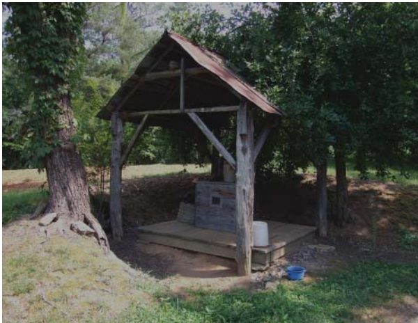
Figure 10. View of Well House in 2008.
