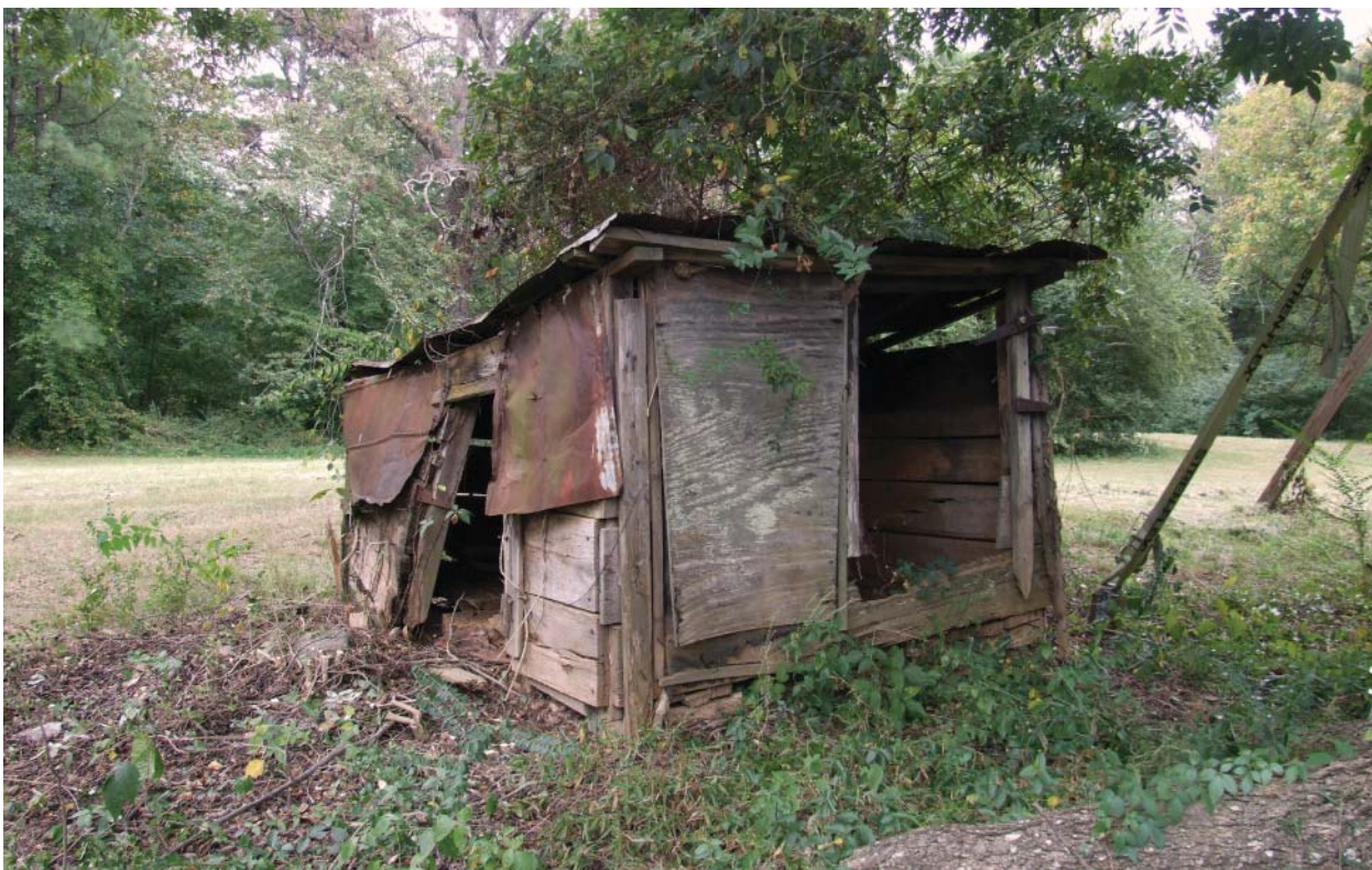
Figure 165. View southeast of Hog House.
