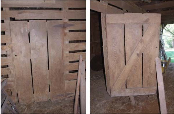
Figure 92. View of door to center crib on east side.
