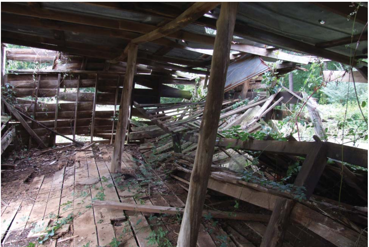
Figure 157. View west in North Chicken House.
