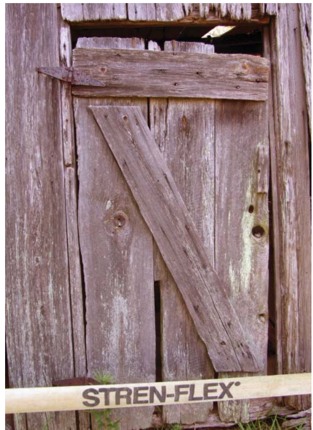
Figure 53. View of door to Old Corn Crib.
