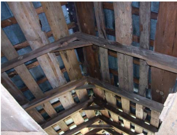
Figure 55. View of roof framing in Old Corn Crib.
