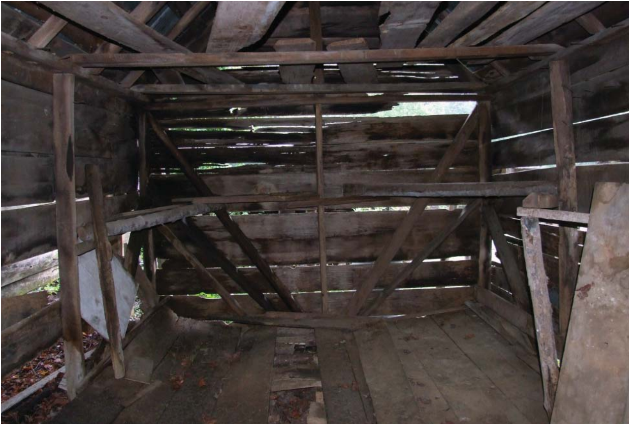
Figure 32. View west inside Gear House.
