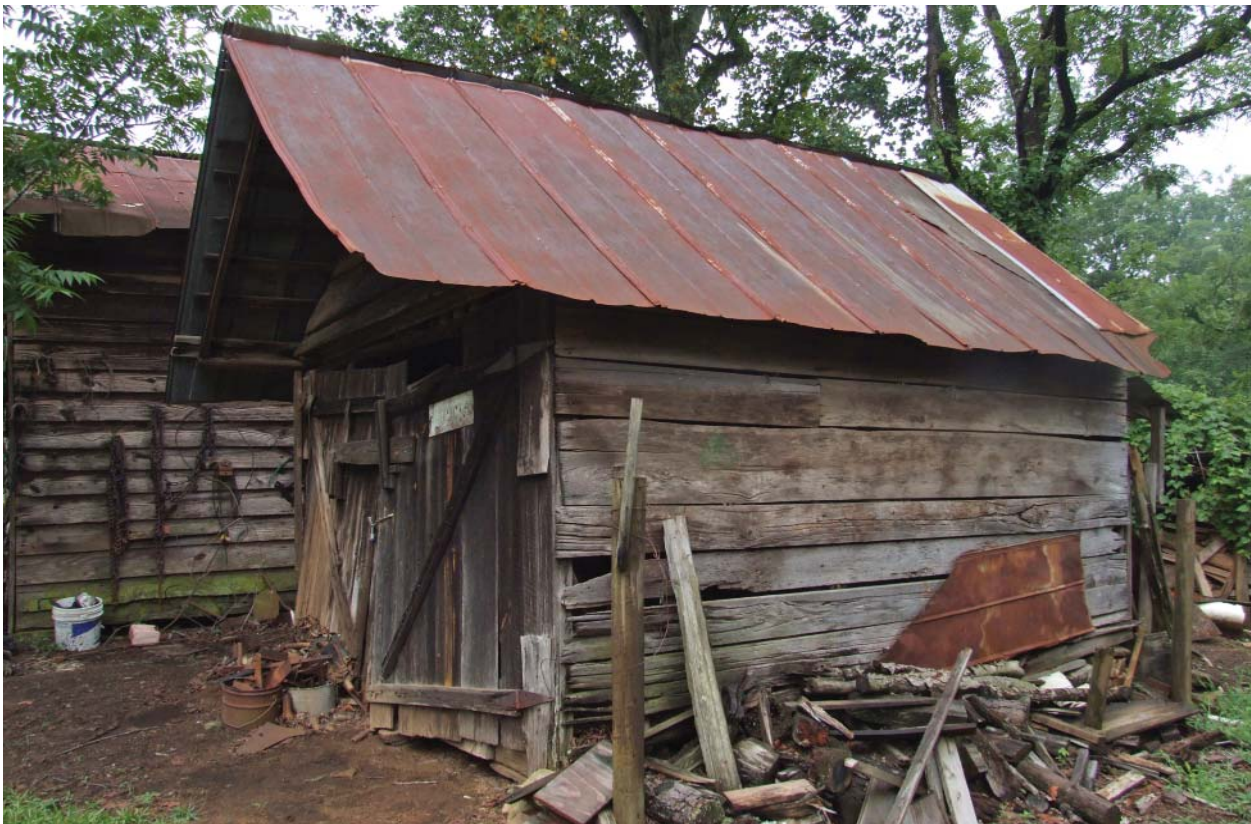
Figure 25 View southwest of Gear House in 2008.
