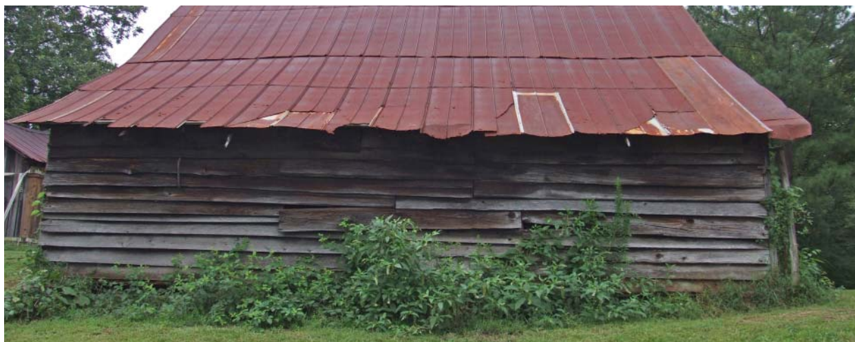
Figure 79. View of west side of West Addition.
