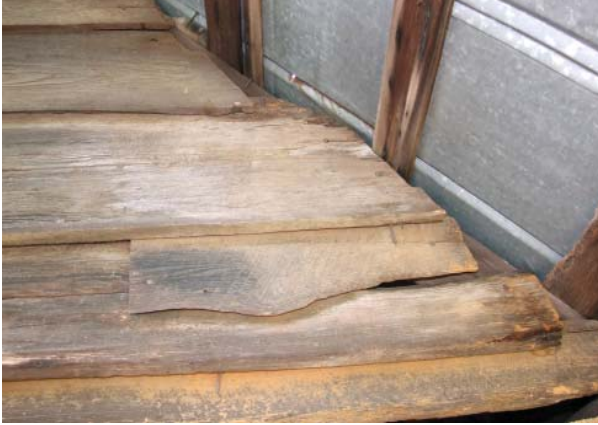
Figure 31. View of siding in front (east) gable of Gear House.
