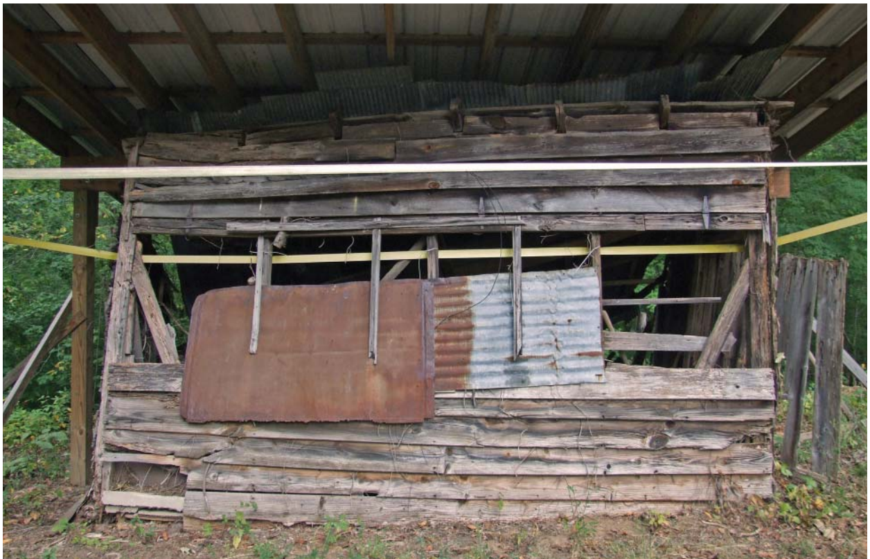
Figure 122. View of front (south) side of Goat House.
