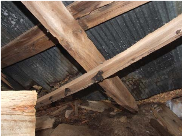
Figure 132. Interior view of roof structure, with interior and exterior purlins visible along with remnants of the tar paper that originally covered the interior.
