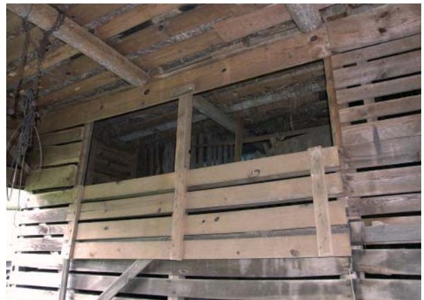
Figure 118. View of drop down doors for loading corn crib.
