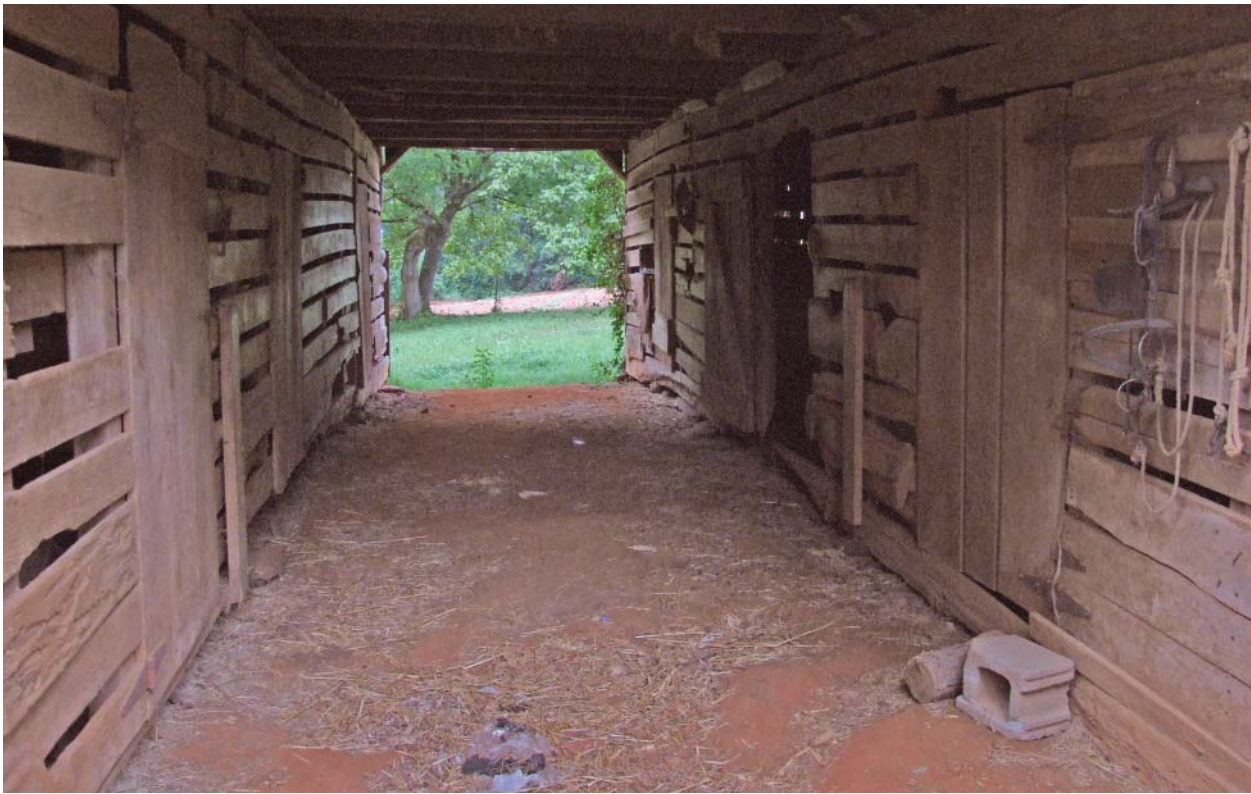
Figure 59. View south of center aisle in the Barn.
