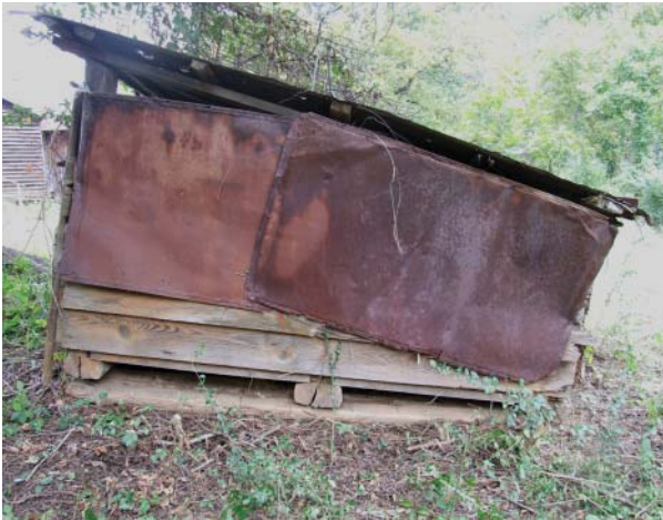
Figure 167. View of south side of Hog House.
