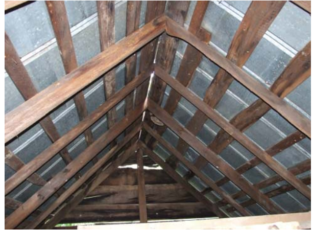
Figure 18. View east of roof framing in Tool Shed.
