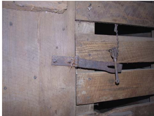
Figure 95. View of metal hasp at door to northeast crib.
