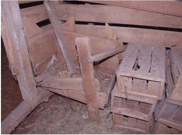
Figure 101. View of floor-mounted trough in southeast crib.
