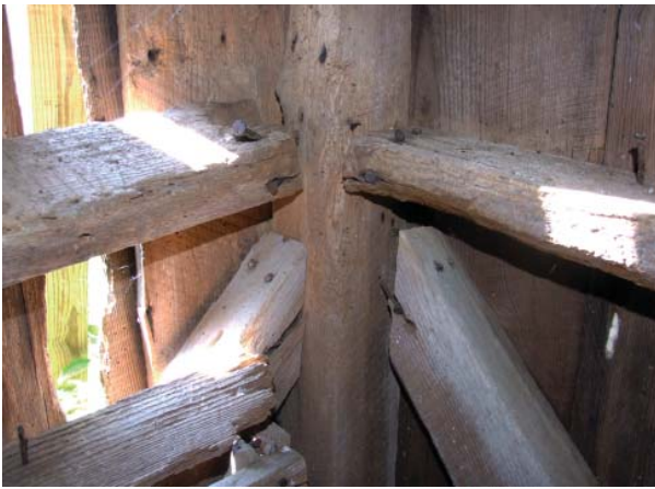
Figure 44. View of typical framing at southeast corner of Old Corn Crib.
