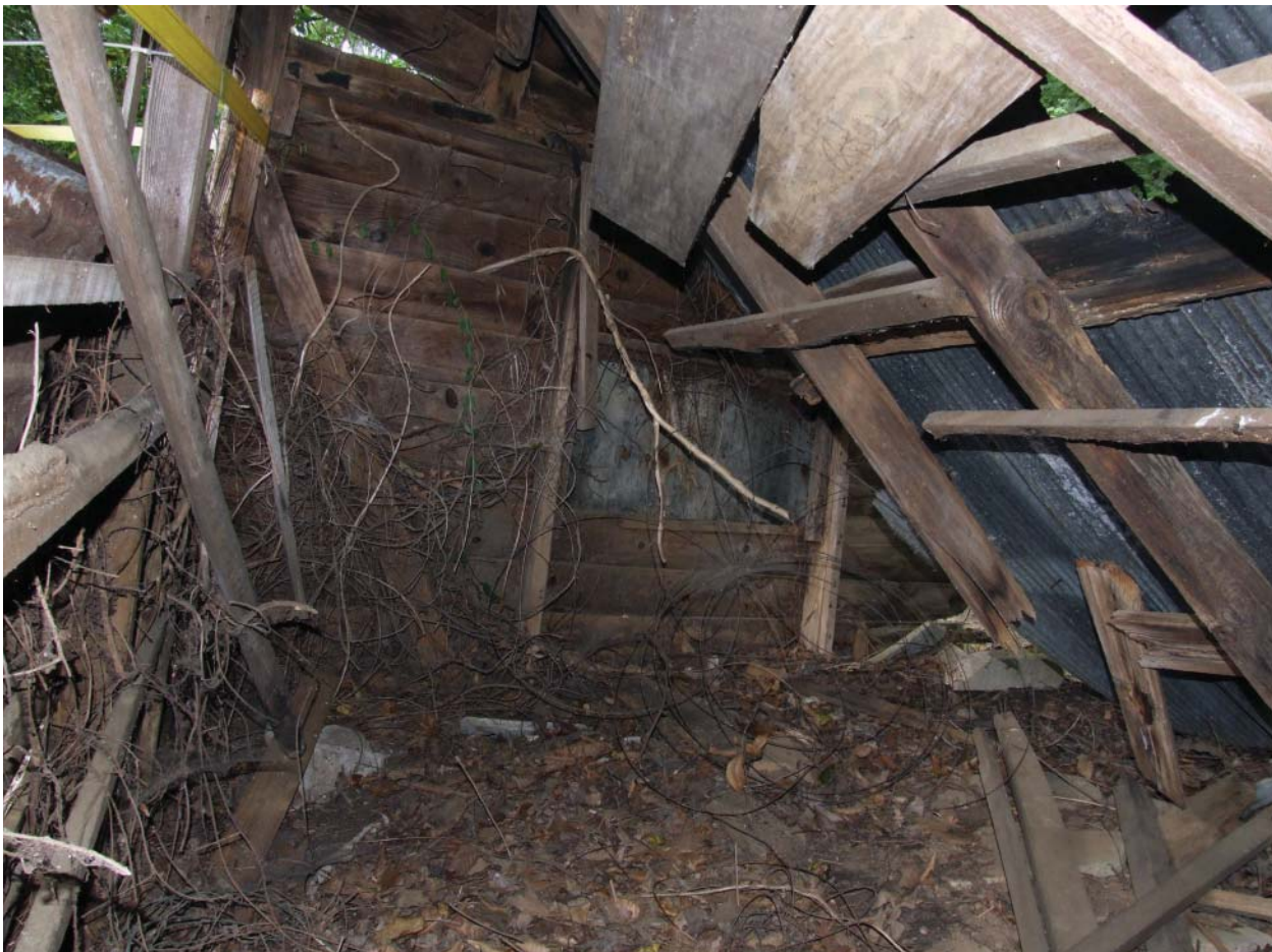
Figure 130. View west inside Goat House.
