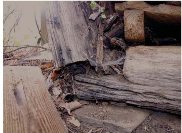
Figure 128. View at northeast corner of Goat House, showing intersection of sills and post, although rot has destroyed most of the sill that lapped over the rear sill seen here.
