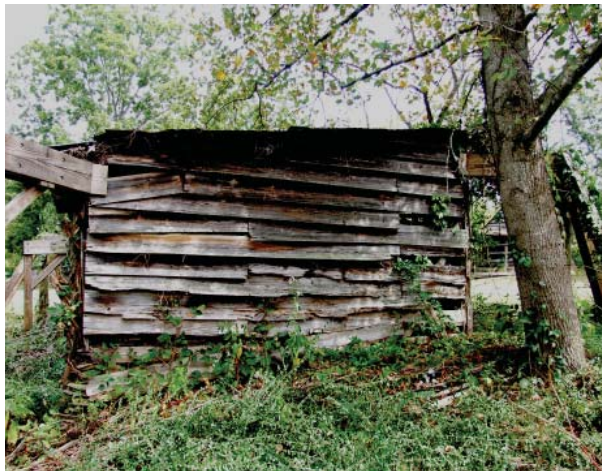
Figure 154. View of west end of South Chicken House.
