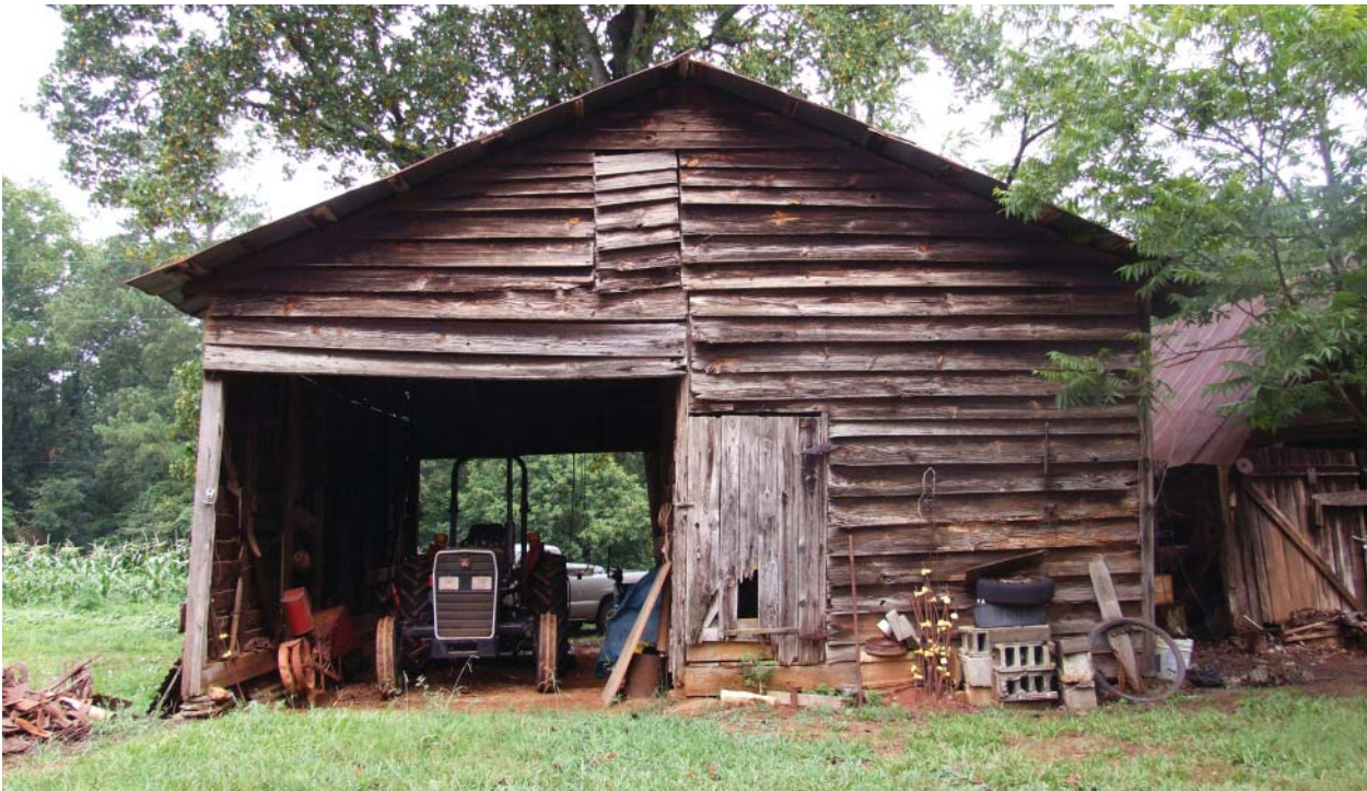
Figure 119. View west of Truck Shelter, left, and Corn Crib, right.
