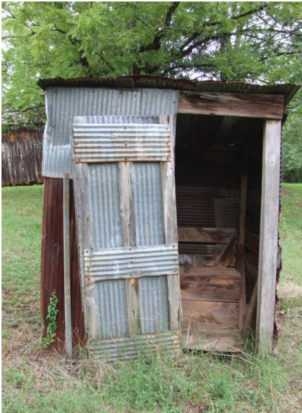
Figure 172. View of front (south) of Privy.
