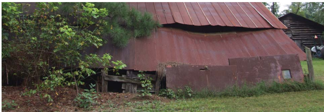
Figure 78. View of exterior of second east addition.
