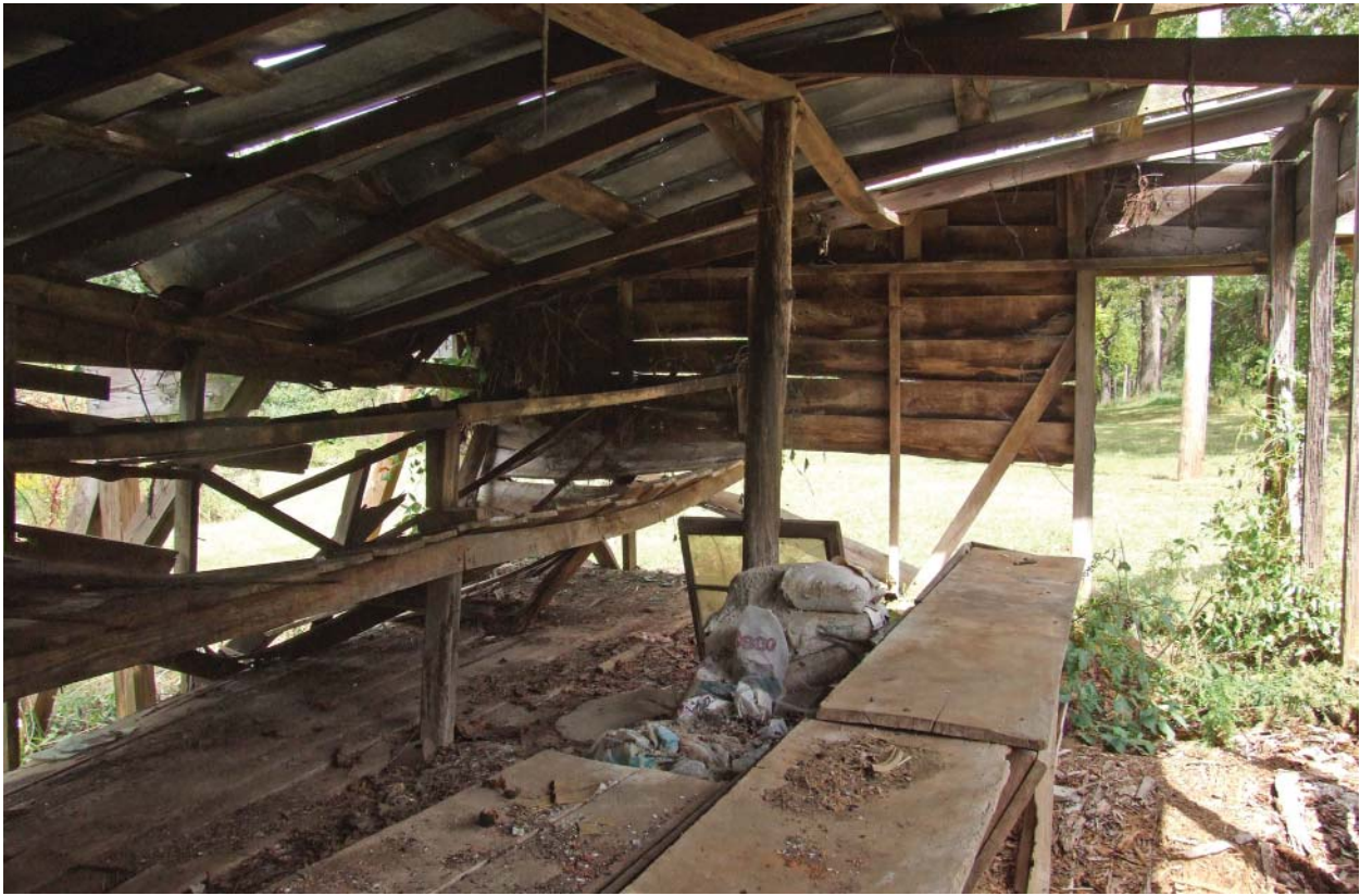
Figure 158. View east in South Kitchen House.
