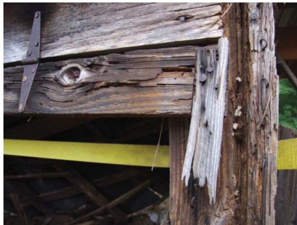
Figure 137. View of east end of front window cover, with remnant of end stile still attached to top rail.
