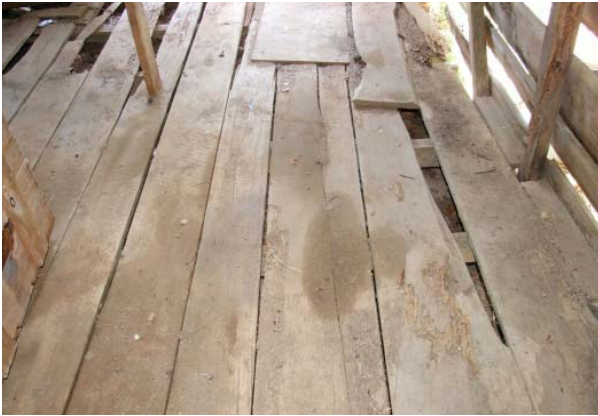
Figure 16. View east of flooring in Tool Shed.
