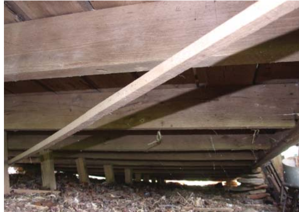
Figure 113. View east of floor framing of corn crib.
