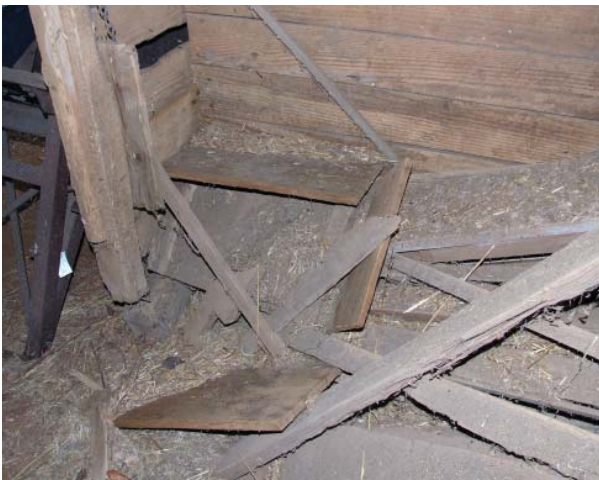
Figure 102. View of remains of feed trough in center crib on east side.
