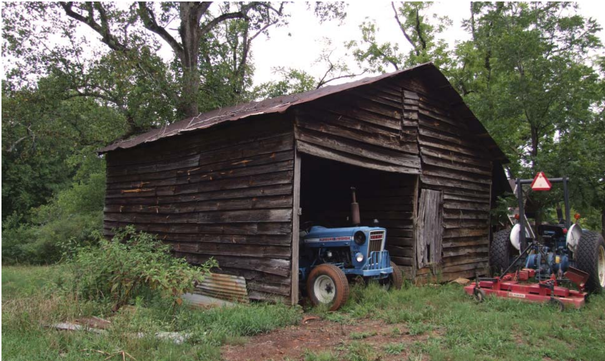
Figure 108. View northwest of Truck Shelter/Corn Crib.
