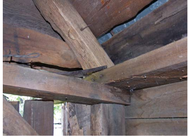
Figure 27. View of framing at southeast corner of Gear House.
