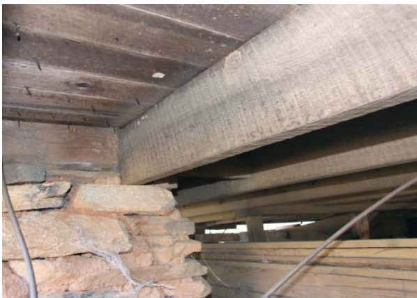
Figure 3. View of circular-sawn joists and flooring in the early twentieth-century additions to the main house. The circular saw blades used to saw lumber were quite large, sometimes over four feet in diameter and marked a very shallow arc in the wood.
