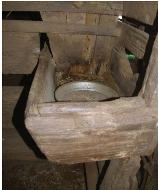
Figure 100. View of trough in middle west crib, which runs through to the next crib.
