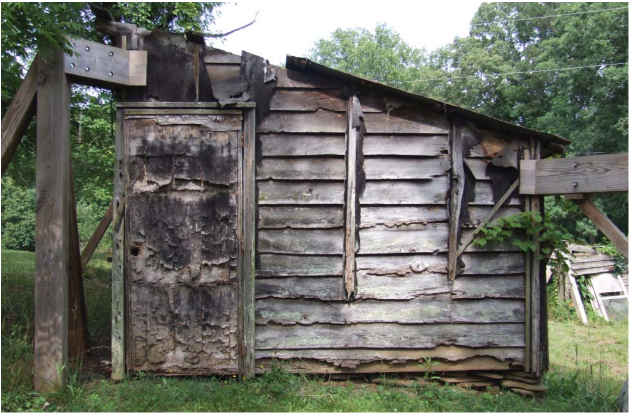
Figure 143. View of east end of Brood House.
