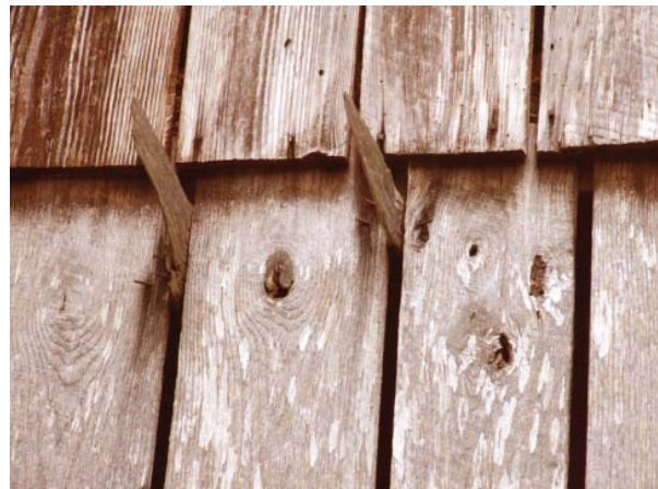
Figure 104. View of what are presumed to be mounts for electrical wiring.
