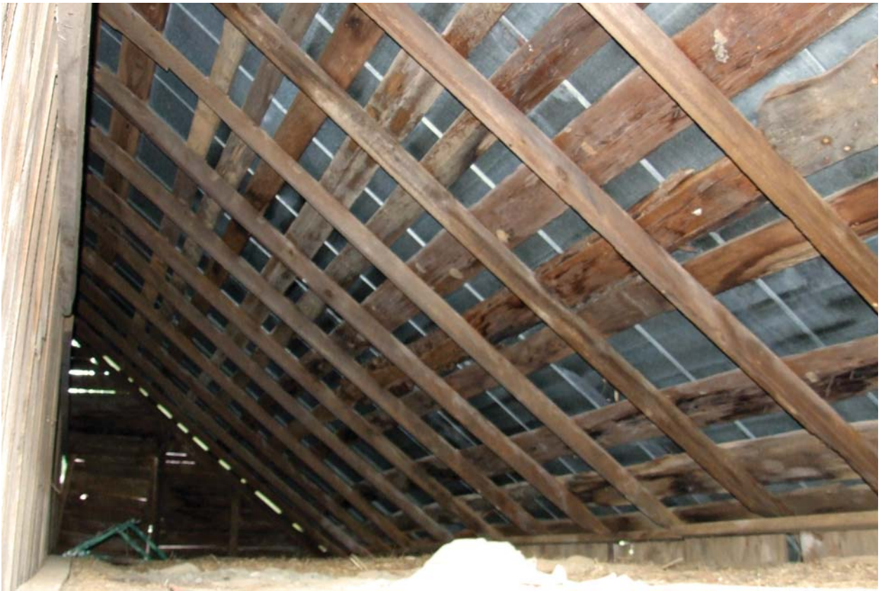
Figure 65. View north in loft of first east addition.
