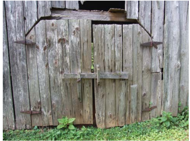
Figure 81. View of doors at front (north) end of center aisle.
