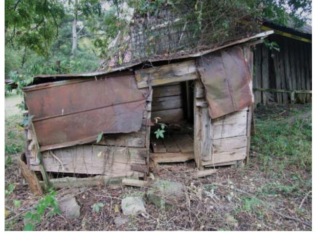
Figure 169. View of north side of Hog House.
