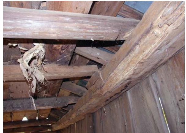
Figure 48. View of typical header, joists, and rafters in Old Corn Crib.
