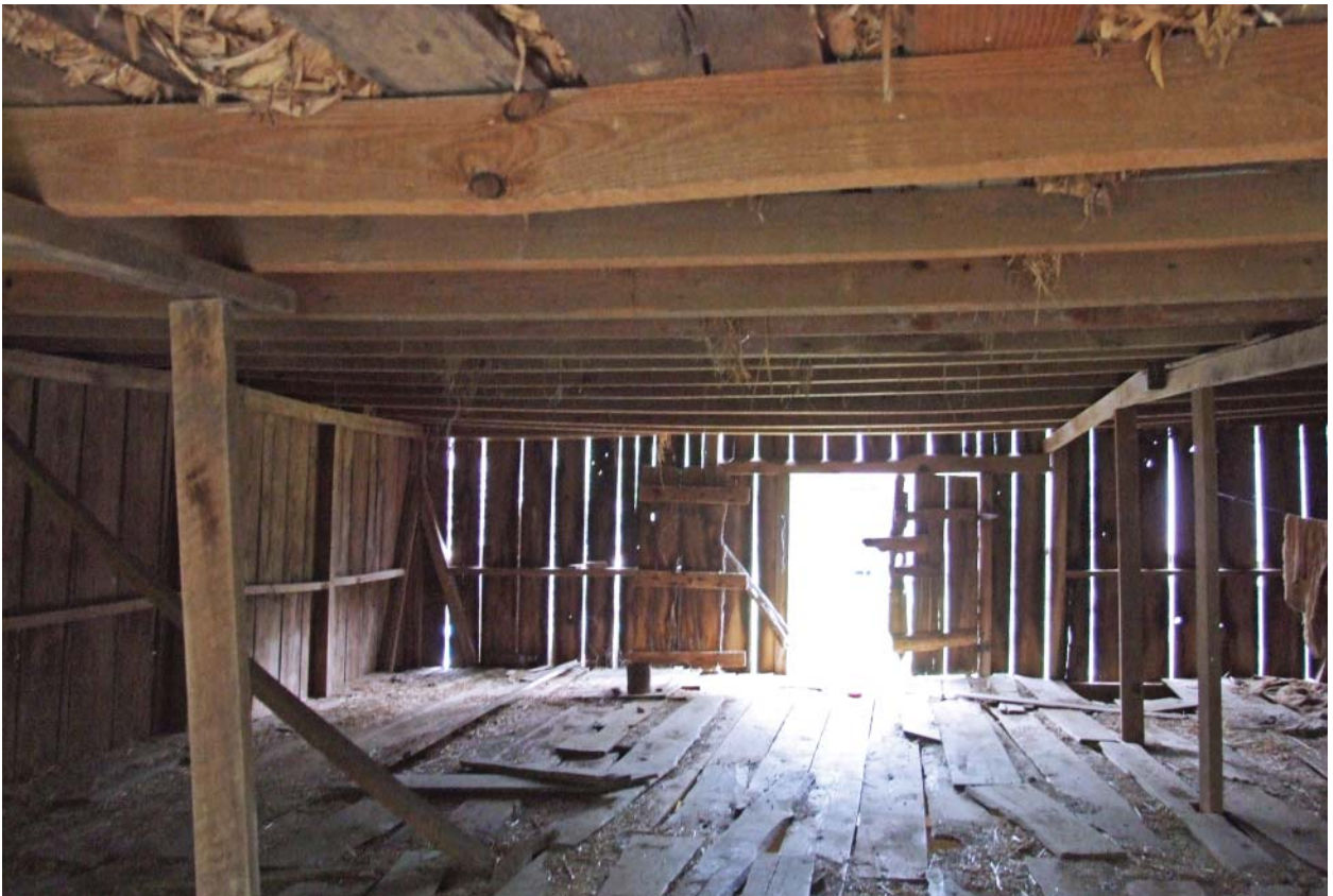
Figure 62. View north in second level of the Barn.
