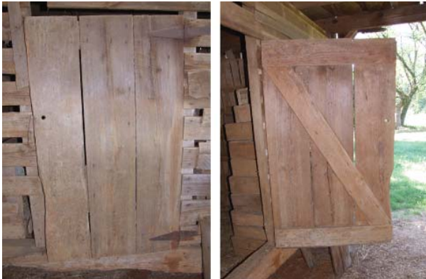
Figure 93. View of door to southeast crib.
