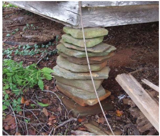
Figure 110. View of rock pier at southwest corner of corn crib.
