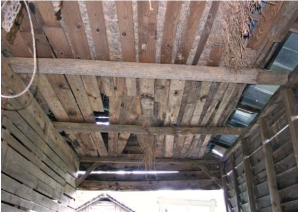
Figure 111. View of log joists for loft over truck shelter.
