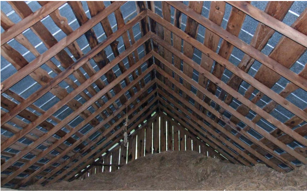
Figure 63. View south in loft or third level of the Barn.
