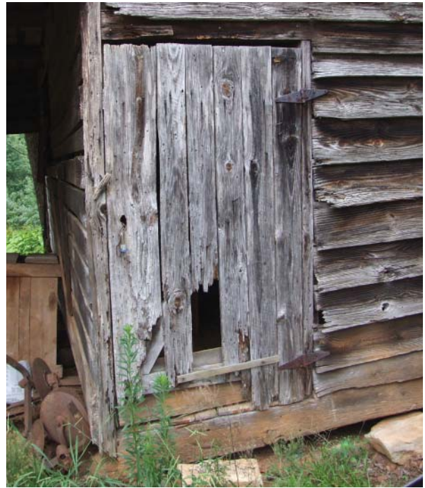
Figure 121. View of door to corn crib.
