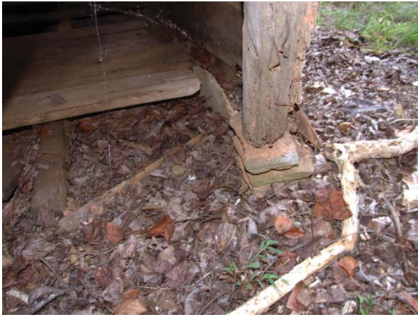
Figure 34. View of southeast corner of Gear House. Note total absence of sills.
