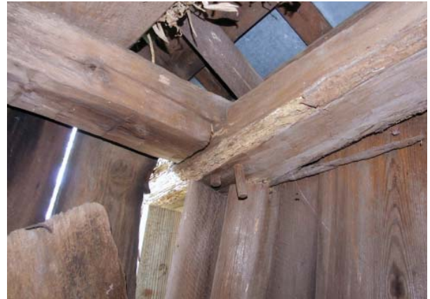
Figure 39. View of wall plates and post at southwest corner of Old Corn Crib.
