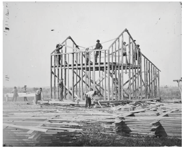
Figure 5. Historic photograph of a balloon-framed building under construction somewhere in the Midwest. (National Building Museum)
