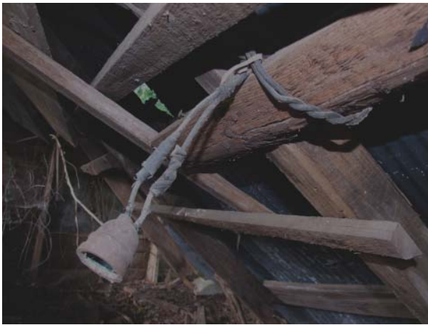
Figure 135. View of Bakelite, keyless socket on interior of Goat House.
