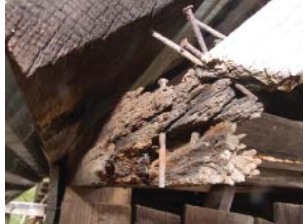
Figure 23. View of end of rafter plate on Tool Shed. Note the mixture of machine cut nails (center) and wire nails.
