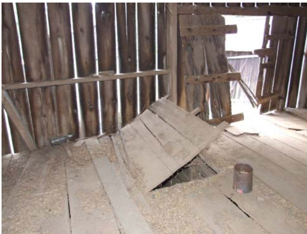
Figure 94. View of trap door above northwest crib.
