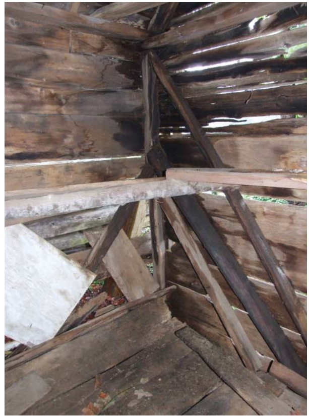
Figure 33. View of bracing at southwest corner of Gear House.
