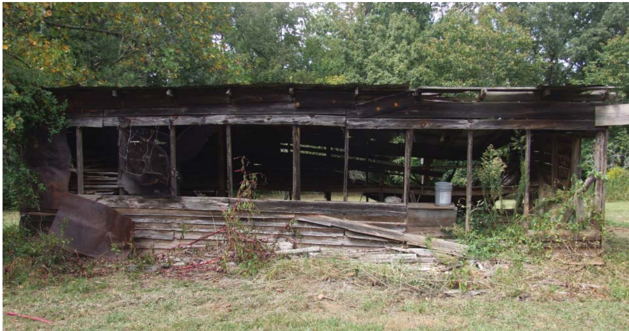
Figure 149. View of front (south) of South Kitchen House.
