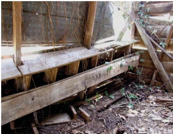
Figure 161. View of nesting boxes along south wall of North Chicken House.
