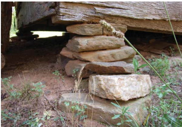
Figure 13. View rock pier at southwest corner of Tool Shed.
