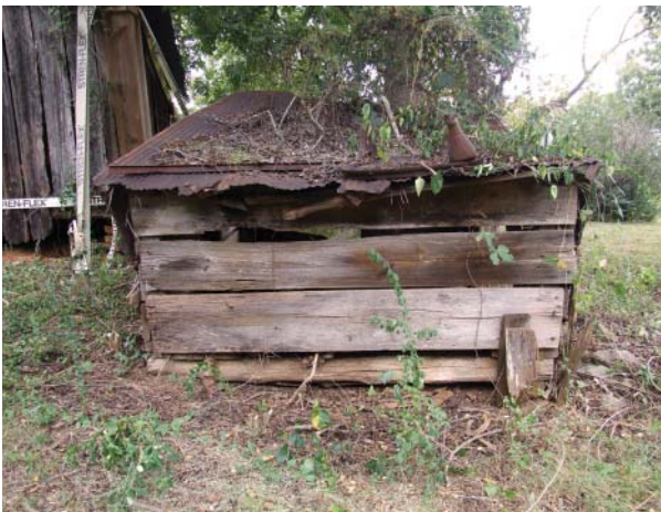
Figure 168. View of rear (east) side of Hog House.
