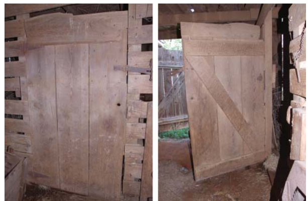
Figure 91. View of door to feed room (northeast crib).
