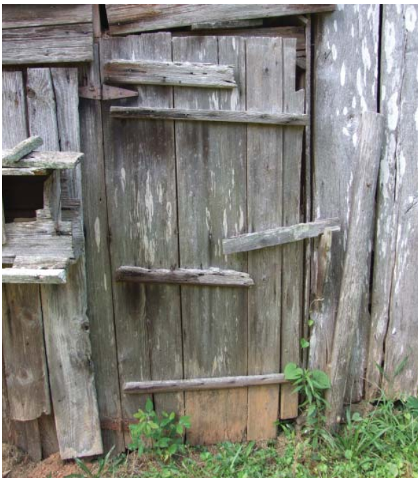
Figure 84. View of door at north end of first east addition.
