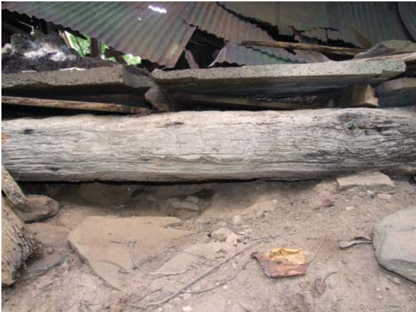
Figure 126. View of rear sill. Ends of floor joists, wood flooring, and concrete overlay are visible..
