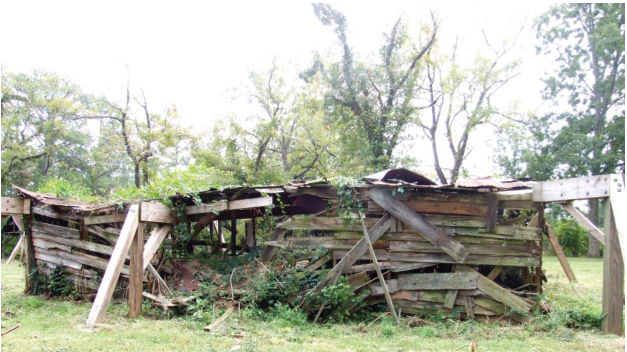
Figure 152. View of rear (north) side of North Chicken House.
