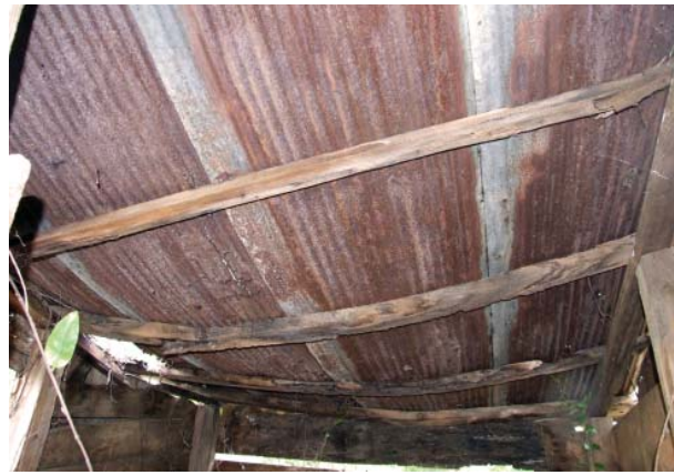
Figure 173. Interior view of Hog House roof.
