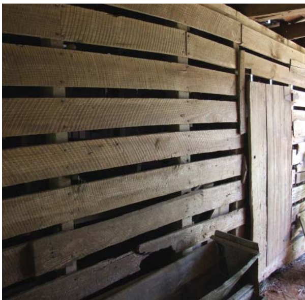
Figure 75. View of board partition typical of both sides of the center aisle.
