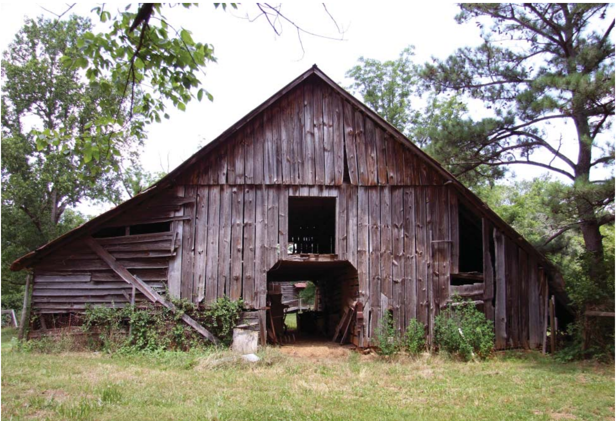
Figure 58. View north of the rear of the Barn.
