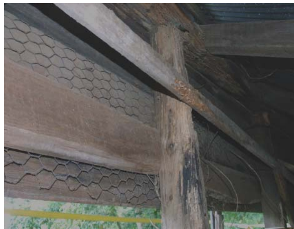
Figure 136. Interior view at top of front window opening.
