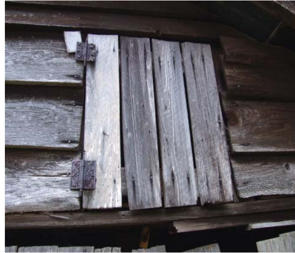
Figure 85. View of loft door at north end of west addition.
