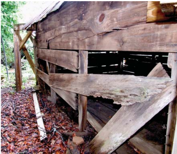
Figure 35. View of south side of Gear House.
