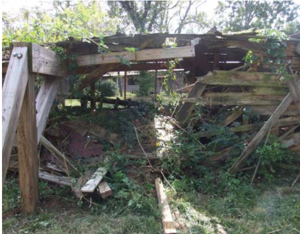
Figure 164. View of rear (north) side of North Chicken House.
