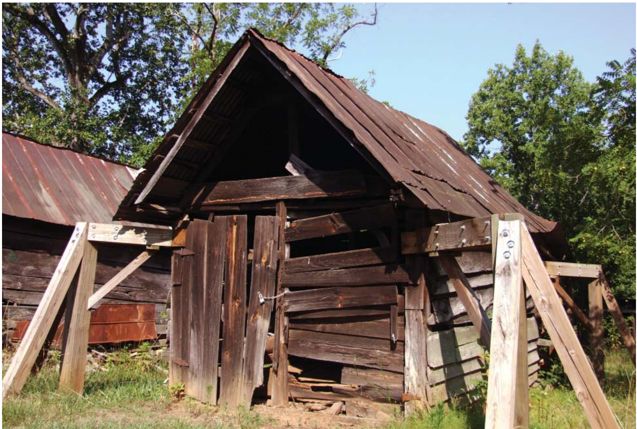
Figure 12. View southwest of Tool Shed.
