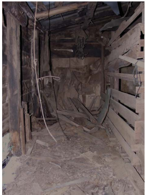
Figure 148. View east along north side of Brood House.
