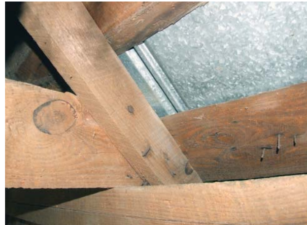
Figure 74. View of typical rafter, joist, and wall plate connection in original portion of the Barn.
