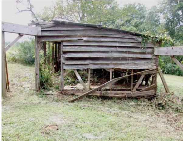
Figure 153. View of east end of South Chicken House.
