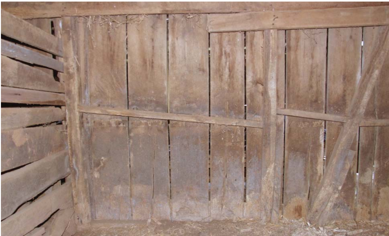
Figure 73. View of northwest stall with typical framing and conditions.
