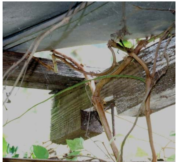
Figure 162. View of typical rafter that was notched to ride over the rear wall plate. A similar detail was used at the front walls of both buildings.
