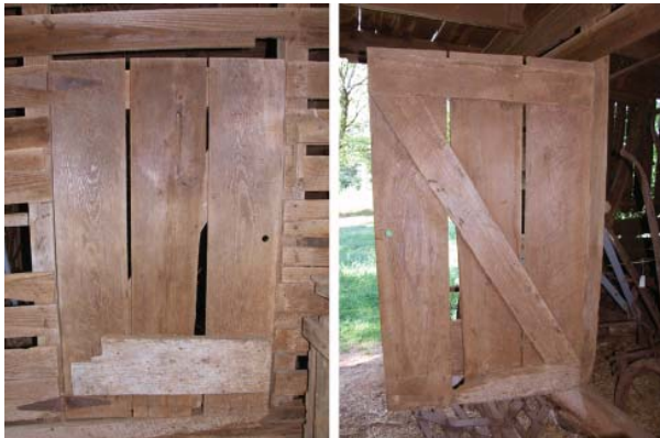
Figure 87. View of door to southwest crib.
