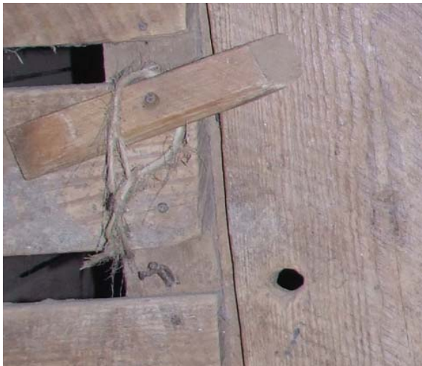
Figure 97. View of typical pivot latch to crib doors.
