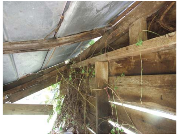
Figure 163. View of framing at northeast corner of South Chicken House.
