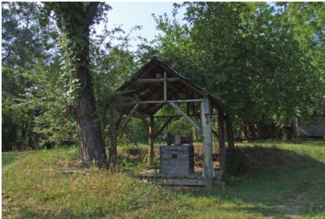
Figure 10. View south of Well House.
