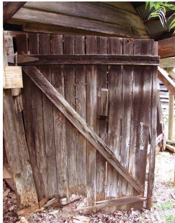
Figure 37. View of one of the doors on the Gear House.
