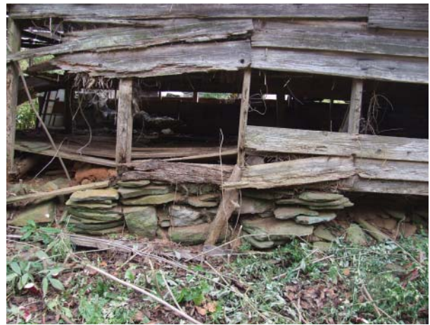
Figure 162. View of rock underpinning at rear sill of South Chicken House.
