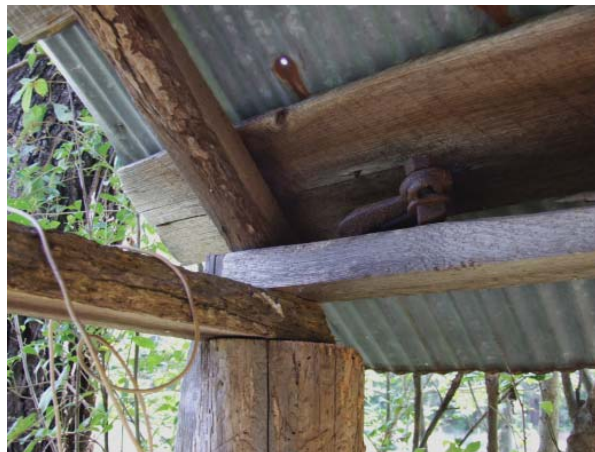
Figure 11. View of framing at northeast corner of Well House.
