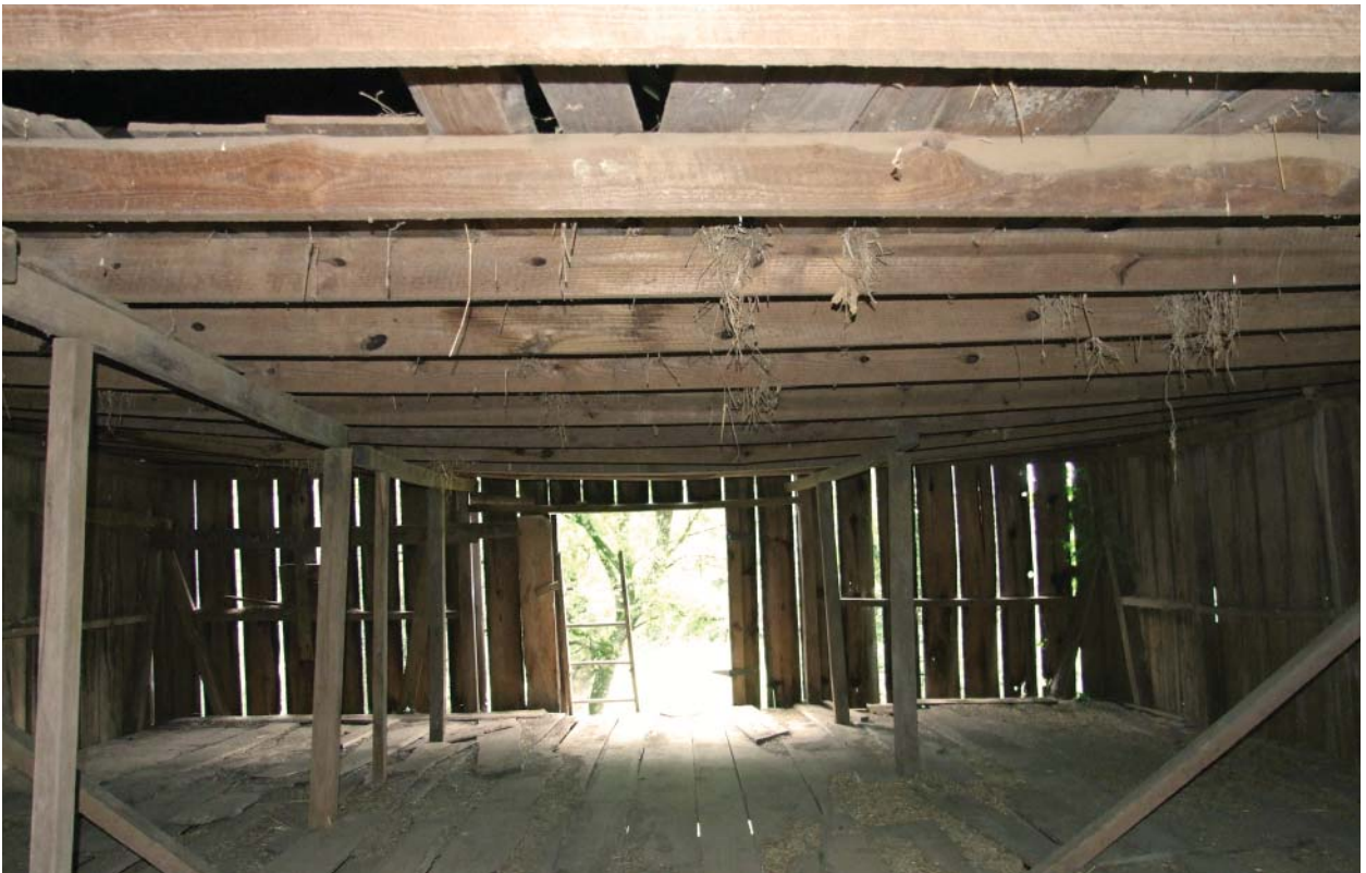
Figure 61. View south in second level of the Barn. Hatch allowing access to loft is at upper left in this image.
