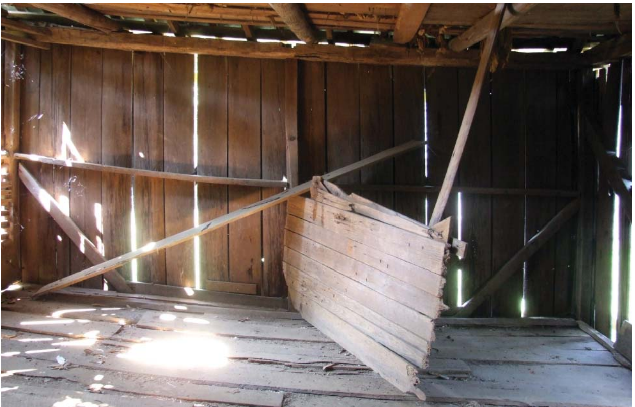
Figure 43. View of south wall with salvaged door nailed to the center post to form a crude partition.
