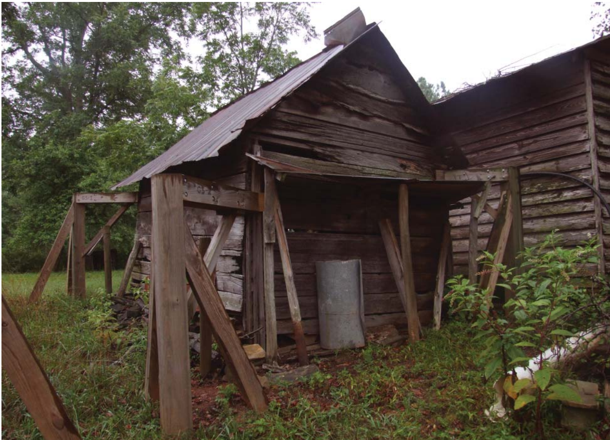
Figure 26. View southeast of Gear House.
