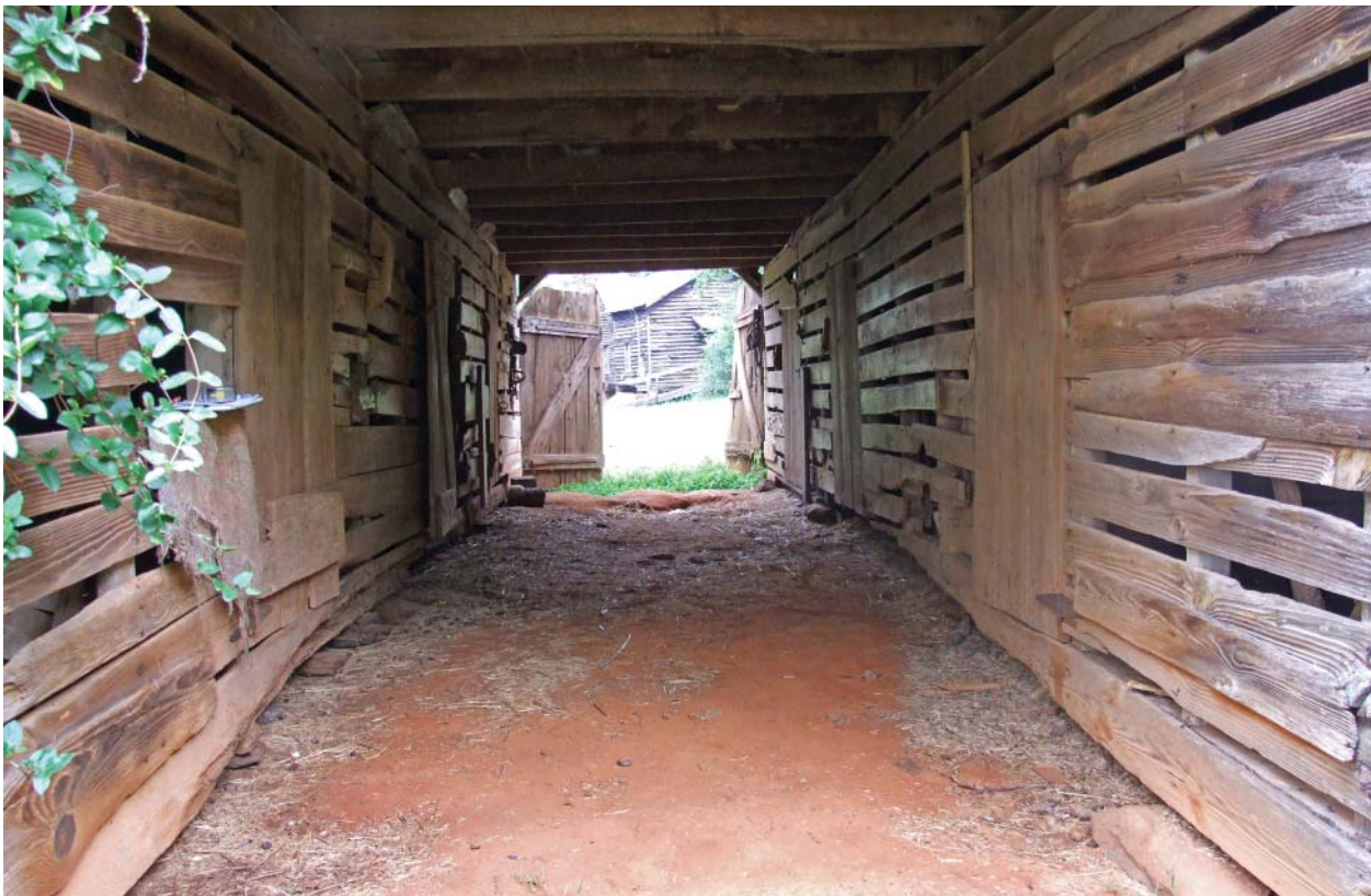
Figure 60. View north of center aisle in the Barn.
