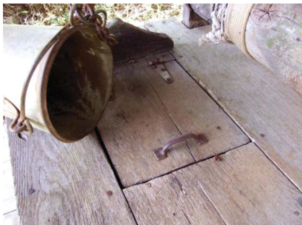
Figure 9. View of top of well cover.
