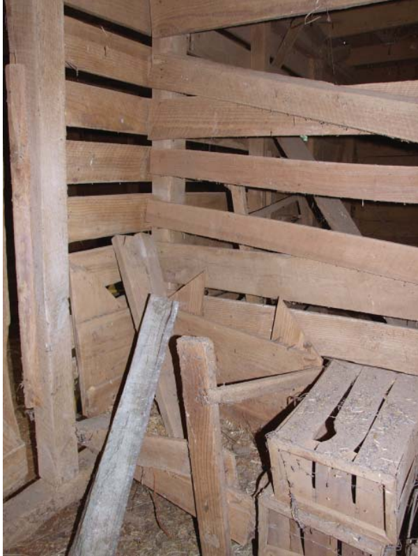
Figure 80. View in northwest crib, with typical partitions between it and the aisle (left) and the adjacent crib (right). Note the broken manger in this corner of the crib.
