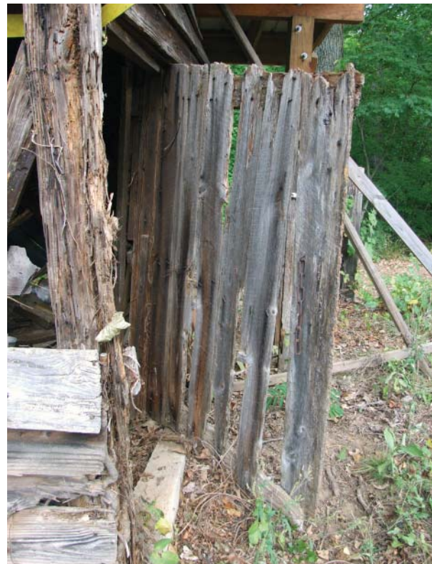
Figure 138. View of inside face of Goat House door.
