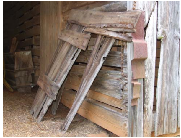
Figure 89. View of what remains of the door to the south end of the loft.
