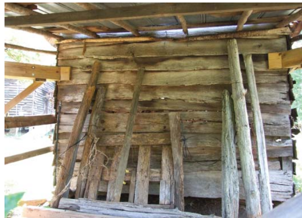
Figure 15. View of rear (west) end of Tool Shed.
