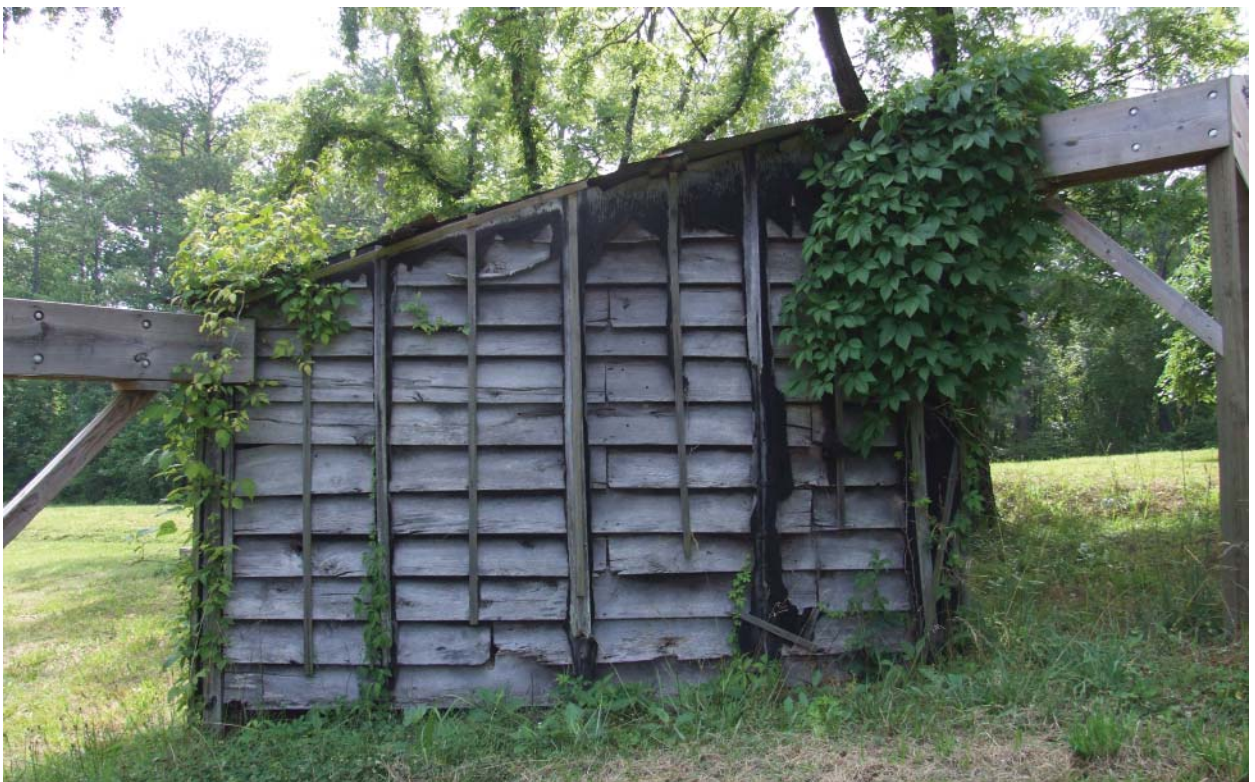
Figure 144. View of west end of Brood House.
