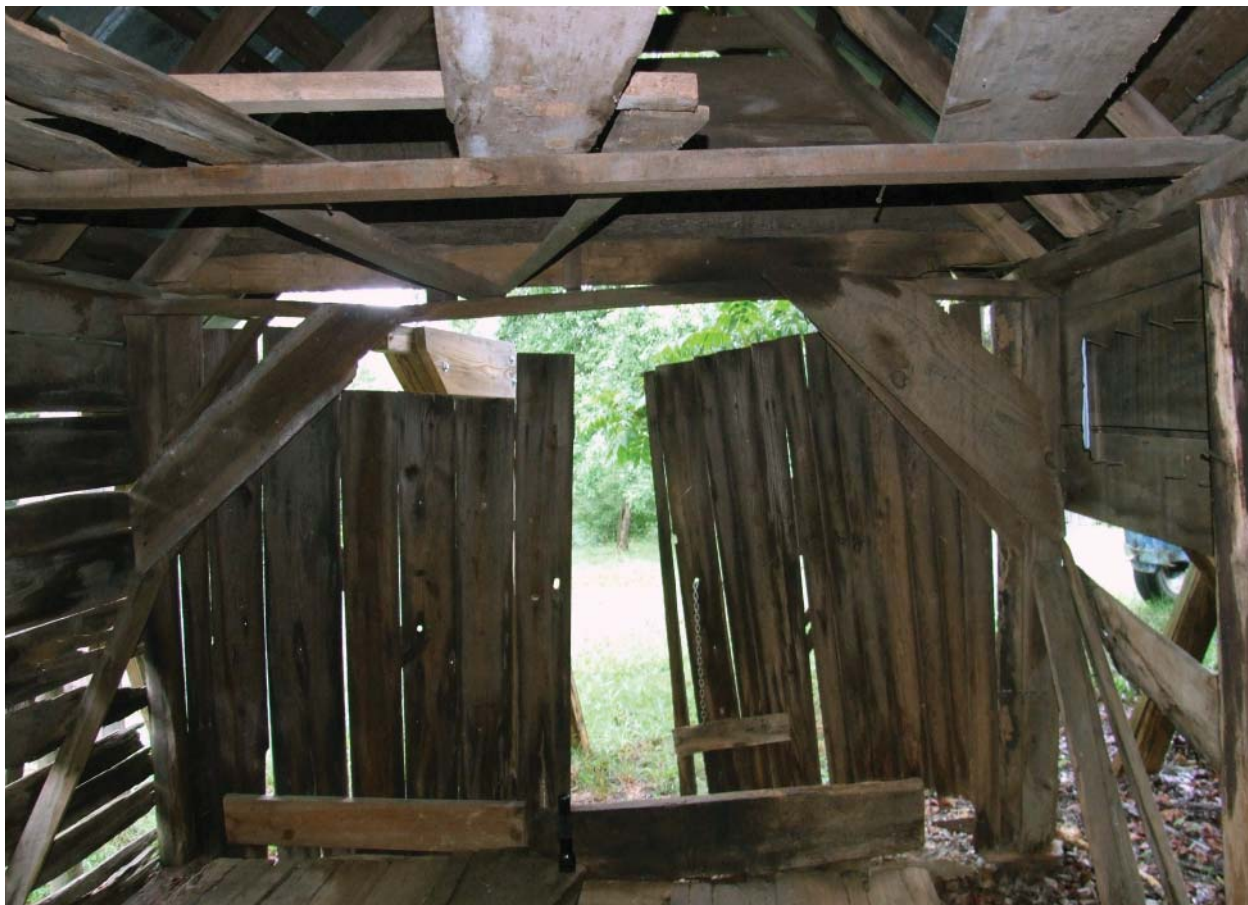
Figure 29. View east inside Gear House.
